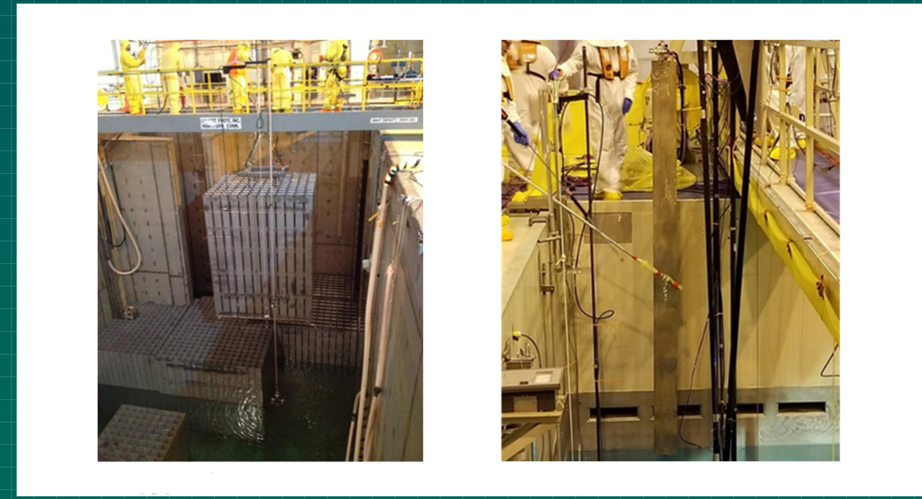
Figure 4 The Zion module is removed from the SFP
