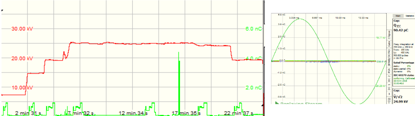
Phase B Time vs. PD / Voltage Profile (FOLLOWING TERMINATION REPAIR)
