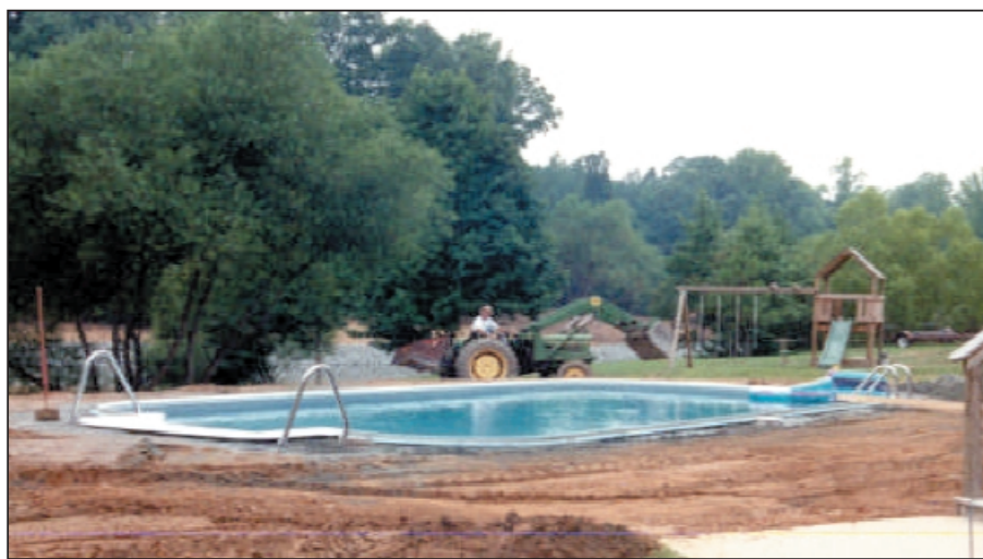
Figure 1. Swimming pool still under construction.
