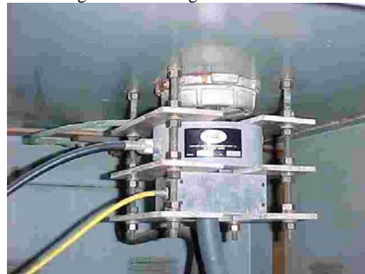
Photo 5. AEP Sensors for Reading EMI. New RFCT Installed Below the Original RFCT.
