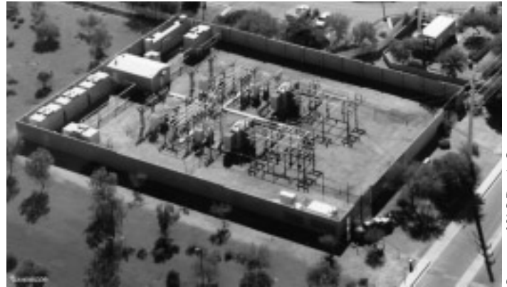
An off-line UPS in a utility substation protects the entire ST Microelectronics semiconductor wafer plant in Arizona, demonstrating how customers and utilities can work together.
