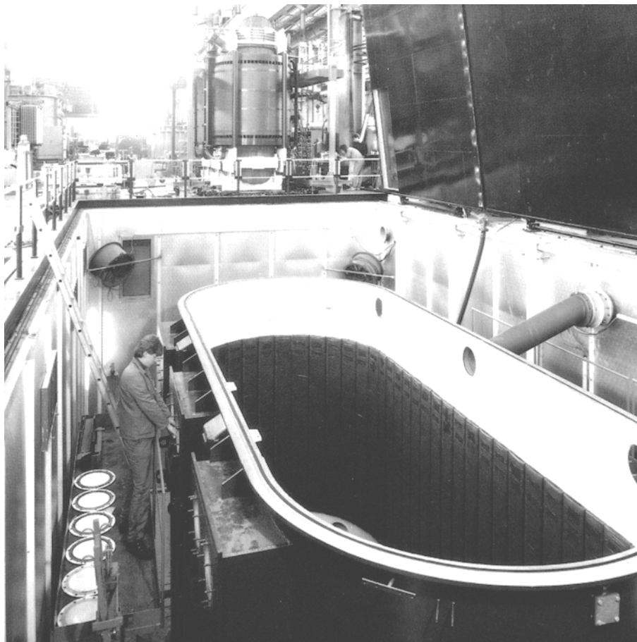
Figure 3-1 Transformer Tank (Courtesy of Smit)
