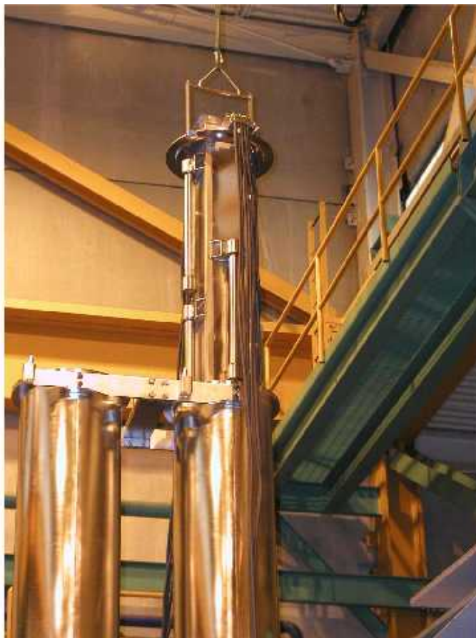
Figure 8-3 STP Transducer Basket Insertion into Reflector Housing
