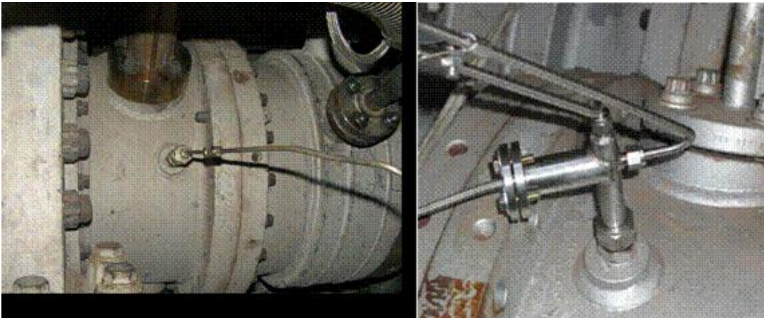
Figure 6-7 Installation of Transfer Tube for Low-Temperature Sensor (on the left) and Installation of a High-Temperature Sensor on GE Combustors
