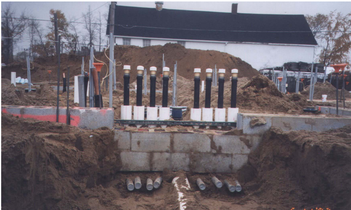
Photograph 2-4 Ground Loop Heat Exchanger Piping Stubouts Installed During Restaurant Construction
