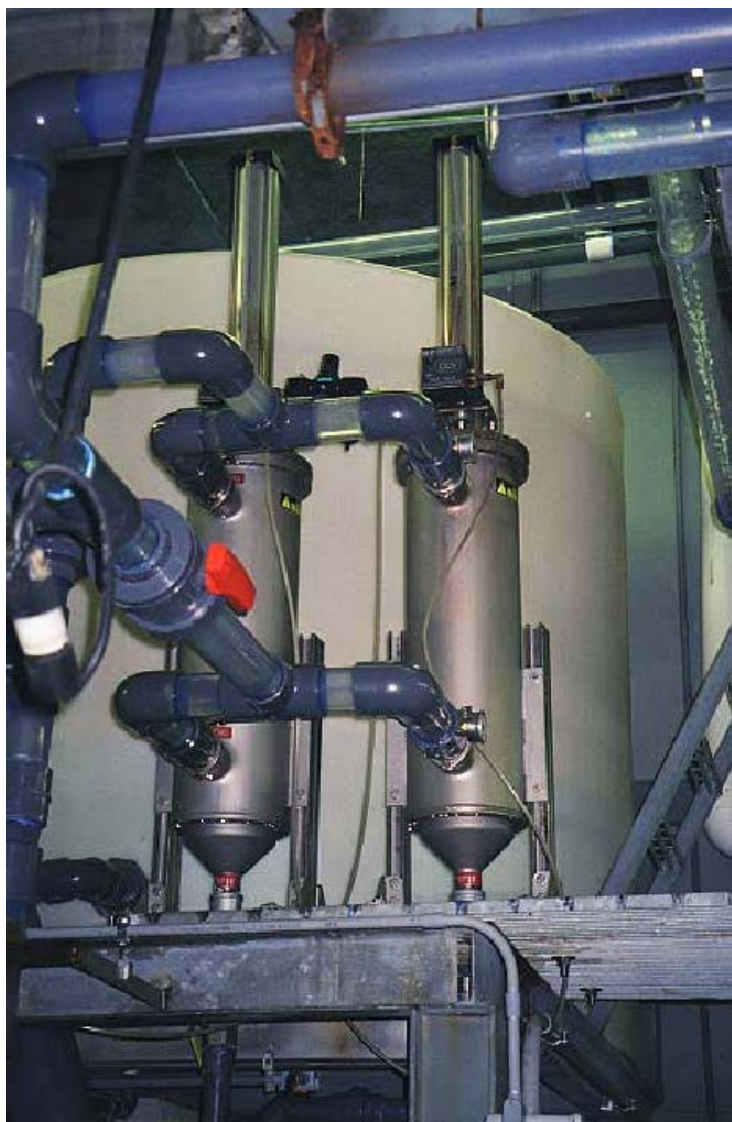
Figure 3-6 The Ronninger-Petter Duplex DCF Filter
