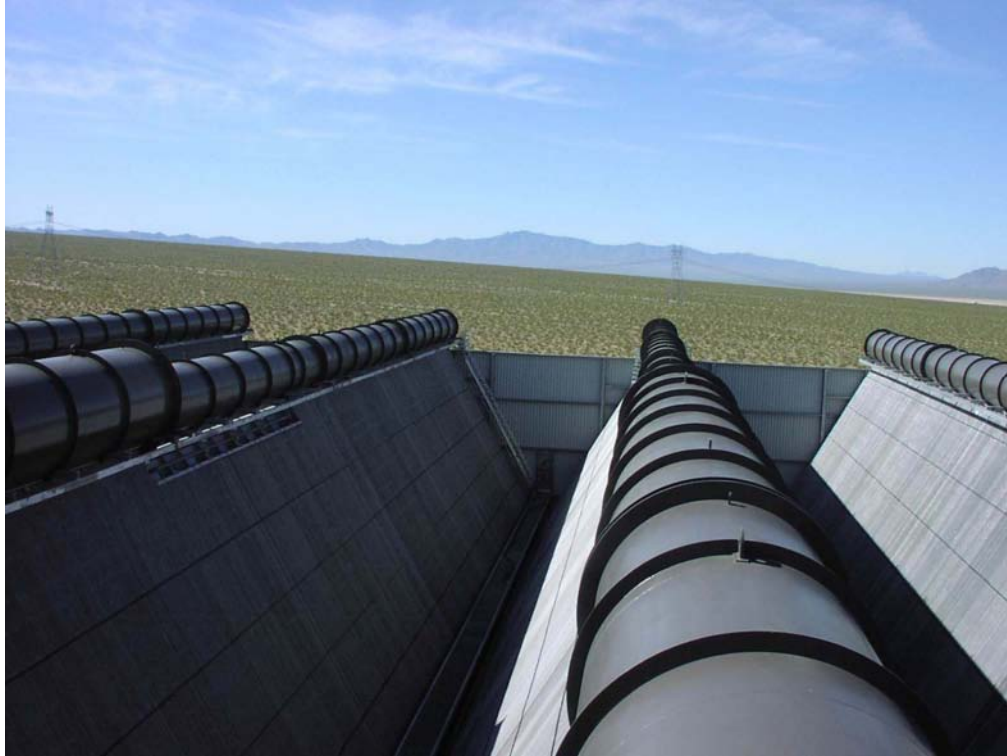
Figure 4-1 Example of Steam Ducting and Finned-Tube Bundles
