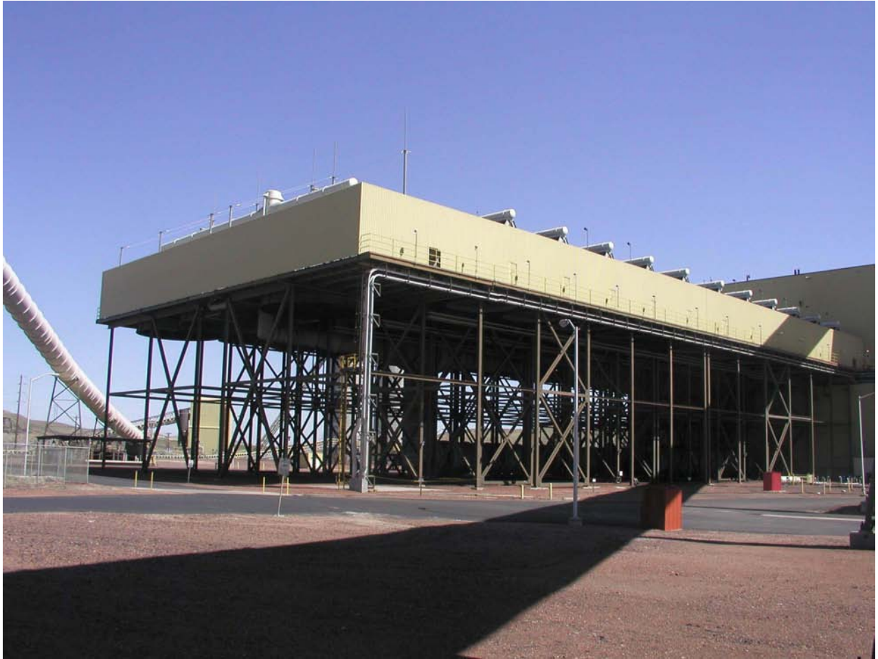
Figure 2-5 Wyodak Air-Cooled Condenser
