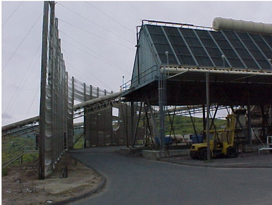
Figure 4-7 Upwind Screen for Reduction of Wind-Entrained Debris and Wind Effects (Chinese Camp Cogen)
