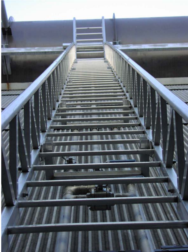
Figure 4-8 Movable Cleaning Ladder System Above Tube Bundles
