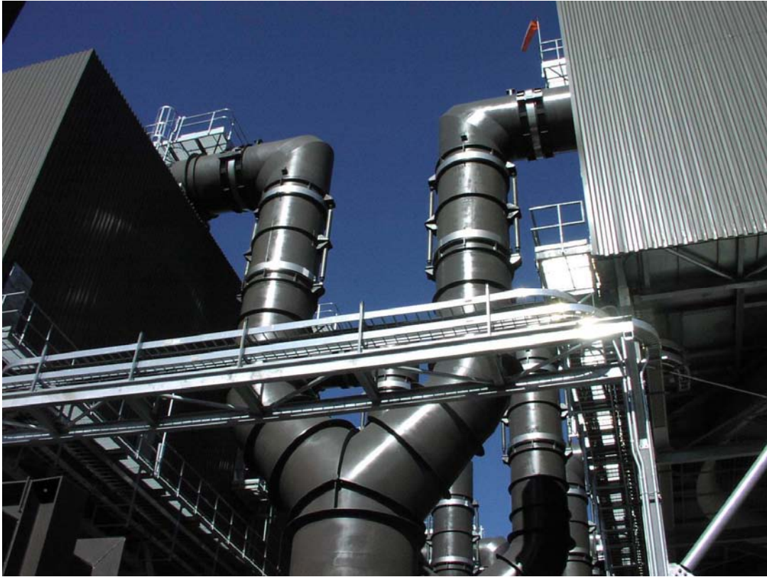
Figure 4-2 Example Steam Ducting and “Pant Leg” Distribution
