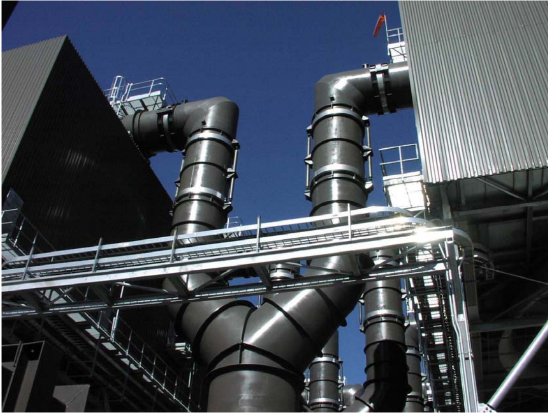
Figure 4-2 Example Steam Ducting and “Pant Leg” Distribution
