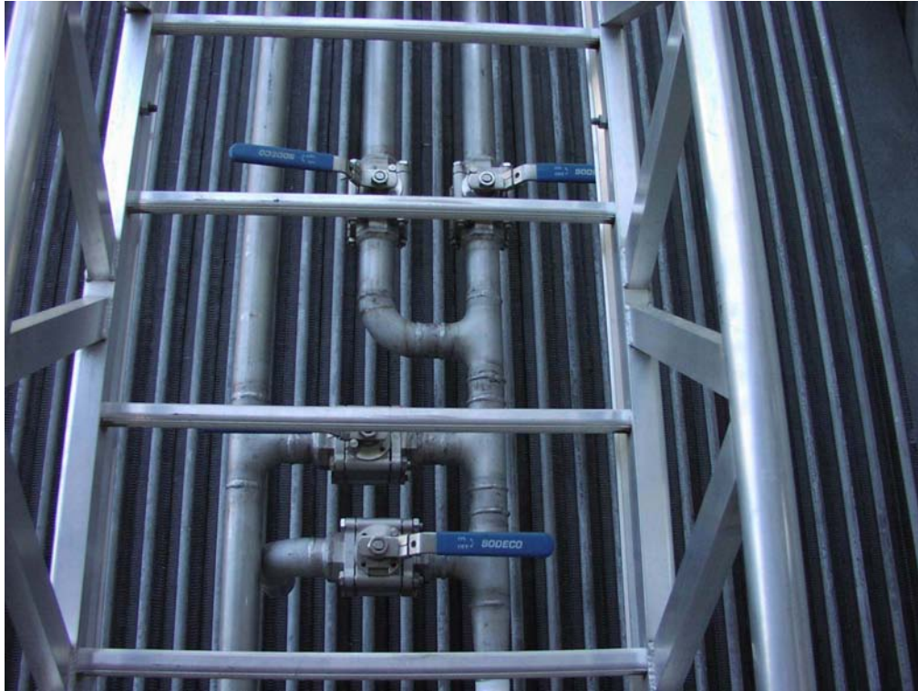
Figure 4-9 Close Up of Spray Cleaner Valving on Movable Cleaning System
