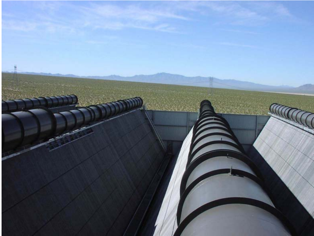
Figure 4-1 Example of Steam Ducting and Finned-Tube Bundles
