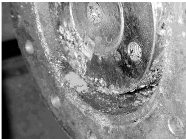
Figure 5-3 Water Infiltration into a Lubricated Coupling Courtesy Rota-Tech Inc.
