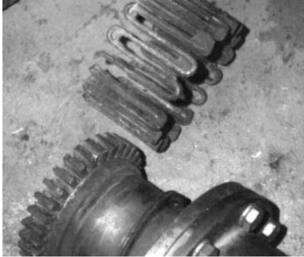
Figure 4-3 Lack of Lubrication on a Grid Coupling Courtesy Rota-Tech Inc.
