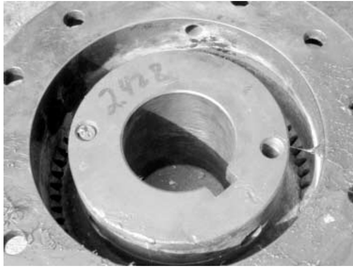
Figure 5-12 Broken Puller Stud Due to Tight Fit on Shaft Courtesy Jack
