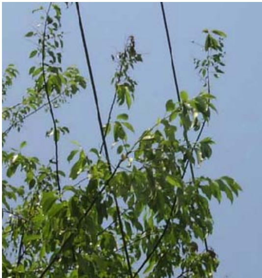
Figure 4-2 Circuits With Impending Tree Growth Contact
