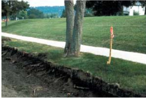
Figure 4-11 Example of Root Damage due to Excavation
