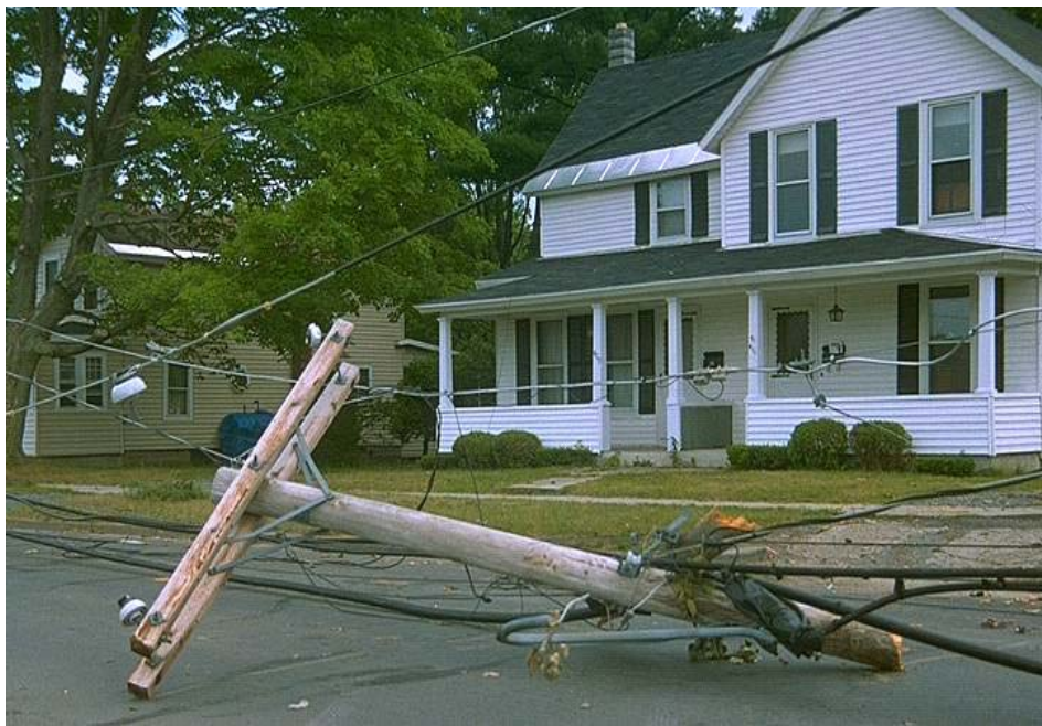
Figure ES-1 A Pole Broken in Half by a Tree Falling onto the Line Structure During a Windstorm
