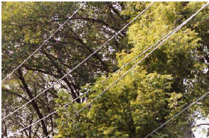
Figure 4-1 Circuits With Significant Tree Overhang
