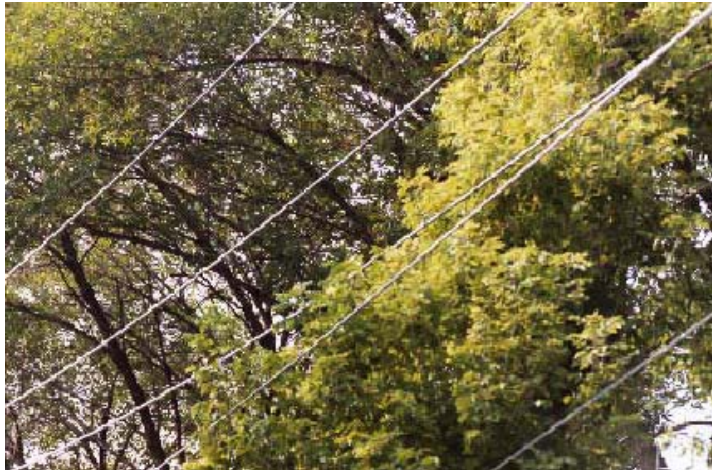
Figure 4-1 Circuits With Significant Tree Overhang
