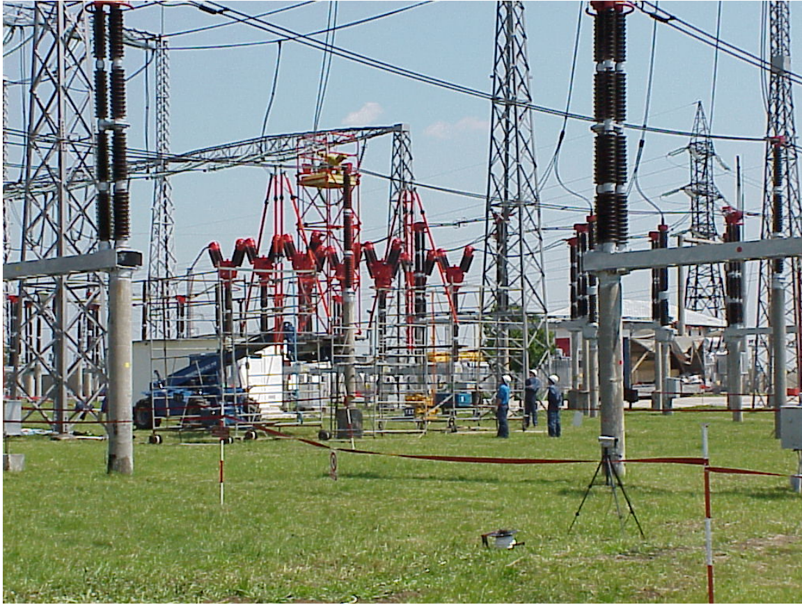
Figure 2-3 Example of scaffolding for maintenance on an energized 400 kV switch.
