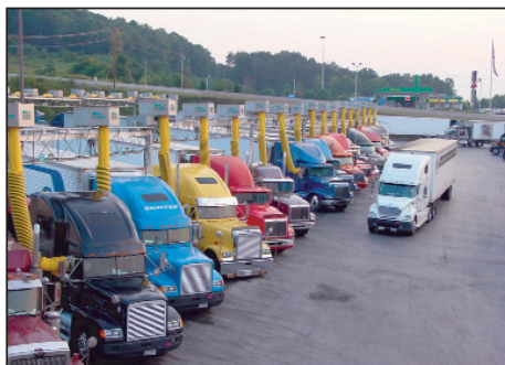
Figure 2. IdleAire TSE Installation.
