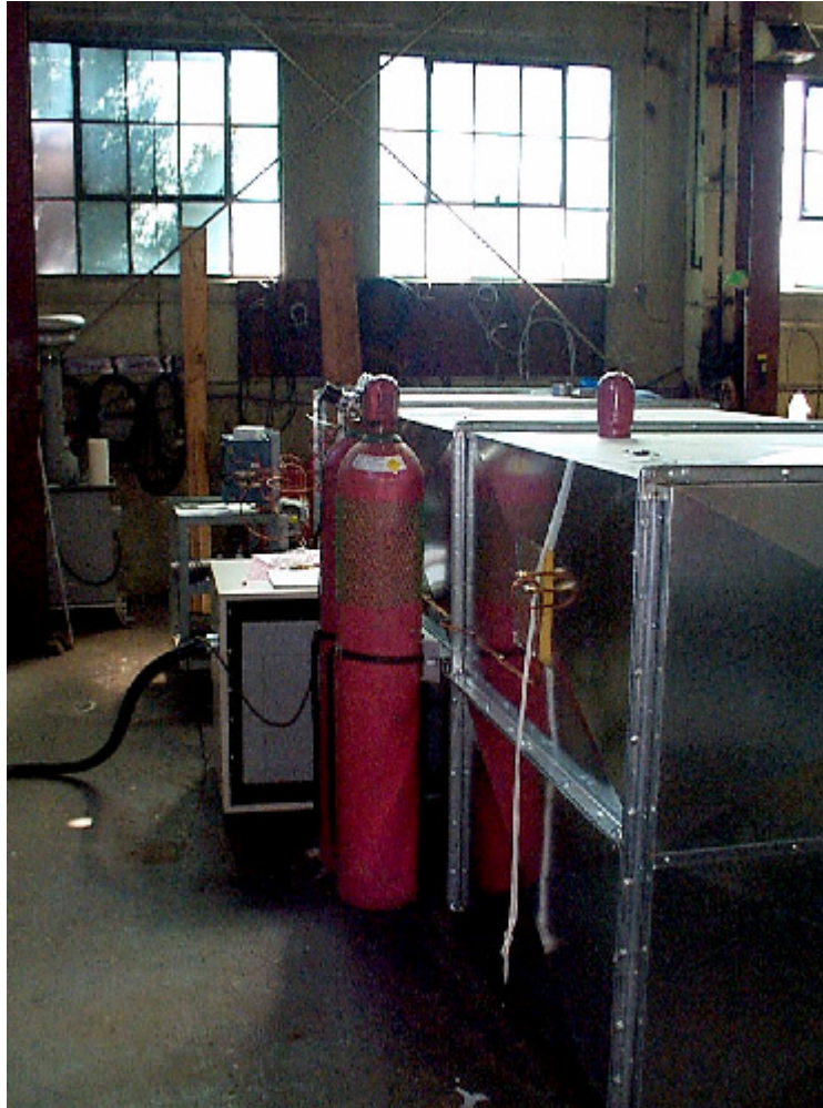
Figure 4-1 View of aging cell with gas handling and temperature control equipment
