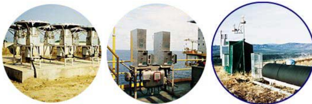
Figure A-6 Global TEG systems providing power for different applications (from left to right: 5,000-W for SCADA, communications and cathodic protection of gas pipeline in India, 200-W TEG for communications and safety equipment in Thailand, and a 100-W unit operated since 1985 for navigational aids in the Yukon, Canada)
