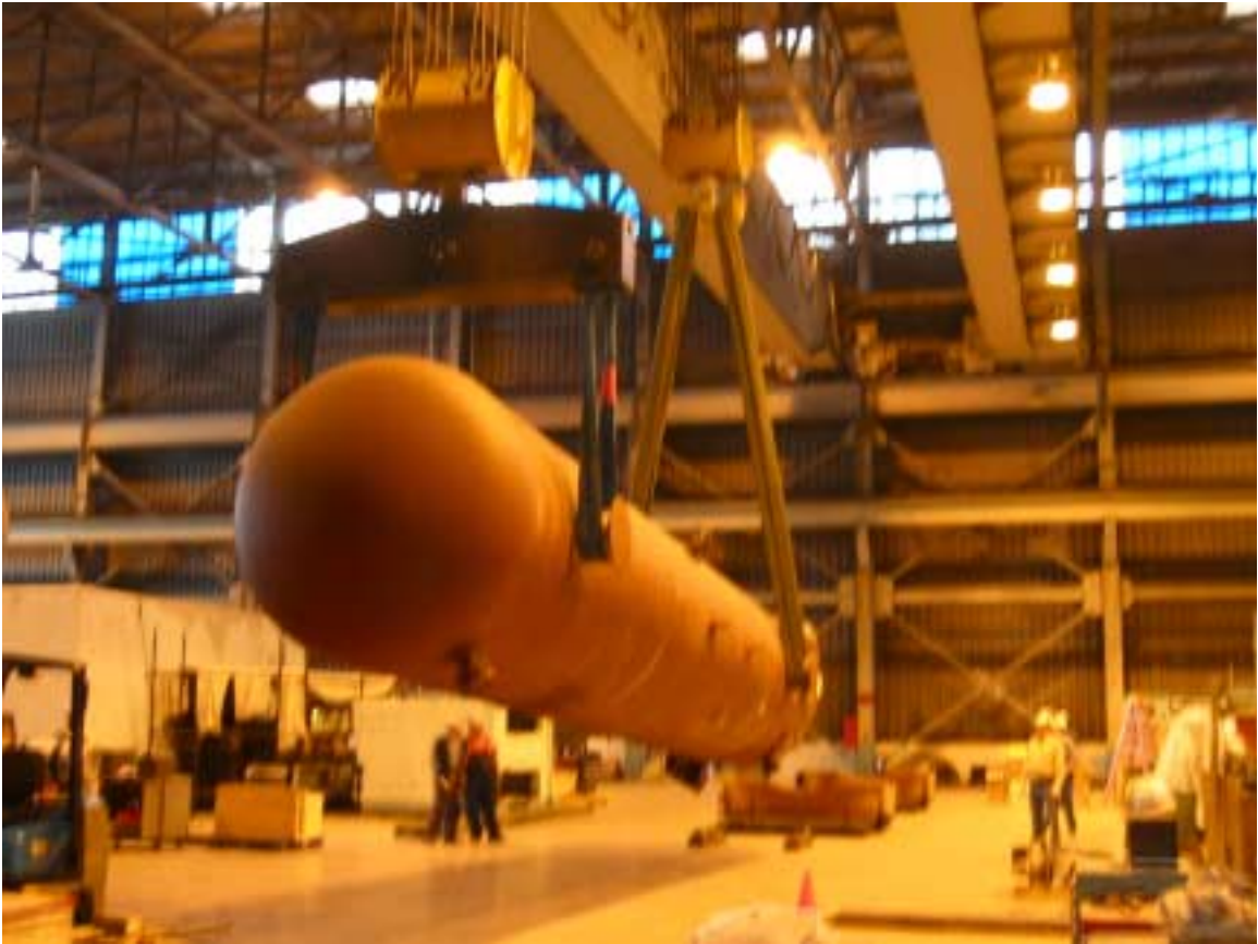
Figure 2 New Feedwater Heater Prior to Uprighting Over Heater Bay
