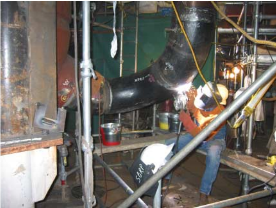
Figure 6 Feedwater Line Welding
