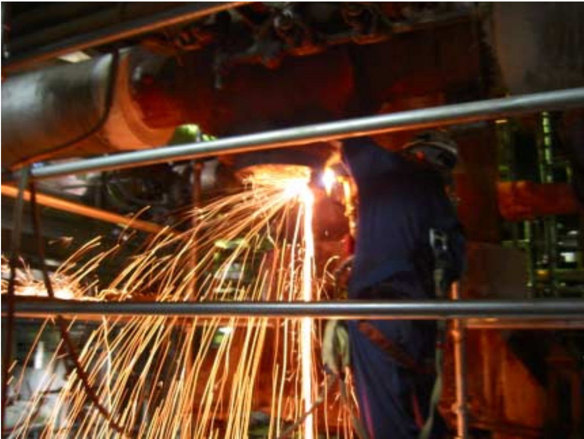
Figure 7 Sparks Fly During Weld Prep/Repair
