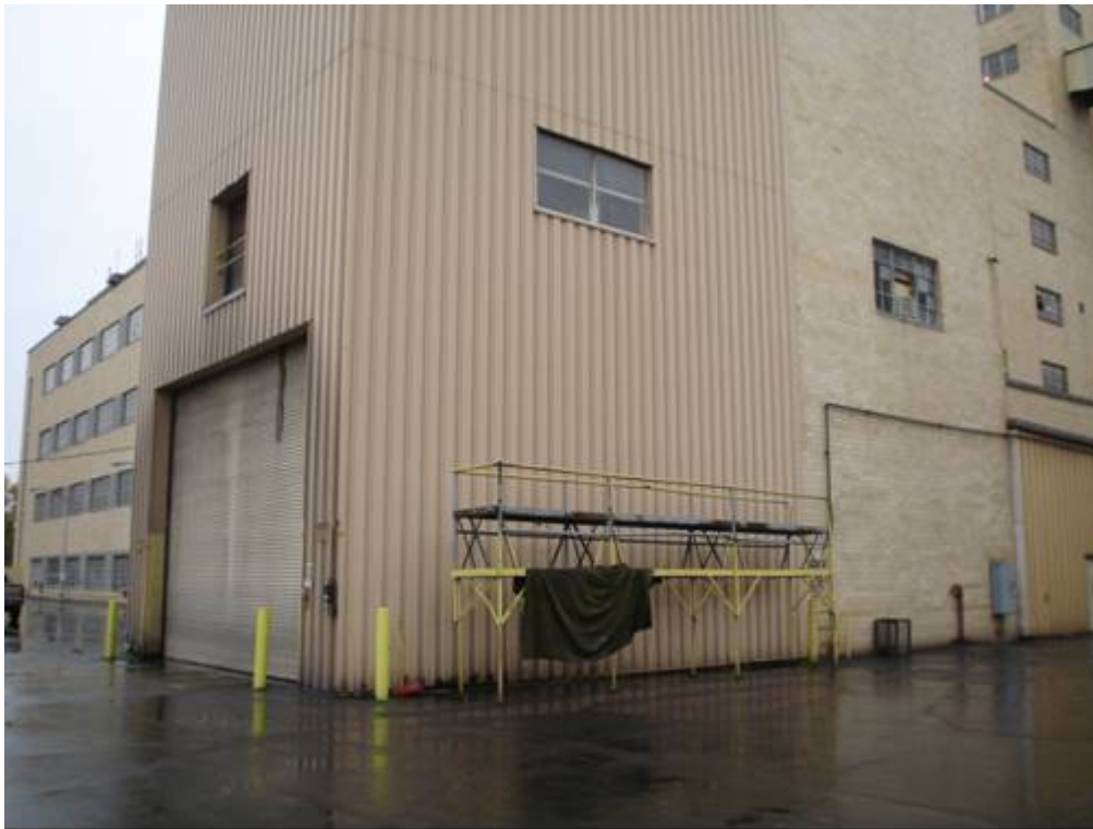
Figure 2-1 Truck Loading Bay for Fly Ash
