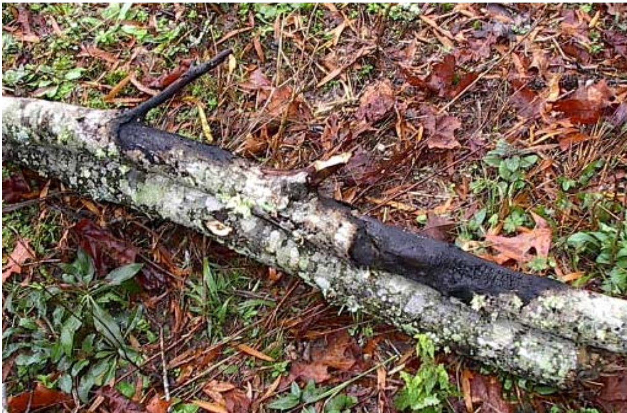
Figure 4-7 Tree Limb that Caused Repetitive Faults and Burned Line Down
