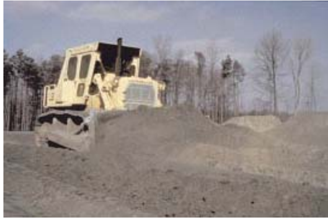
Figure 7-1 Spreading and Compaction of Fly Ash Structural Fill
