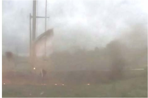
(b) Cover and its frame are ripped off the M11 manhole roof slab and hurled upwards.
