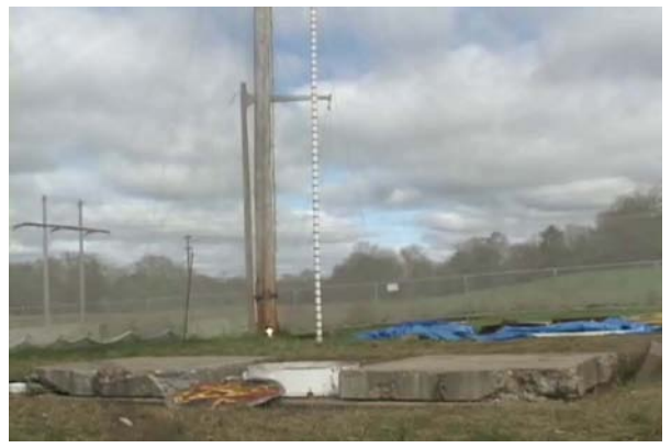
(d) Cover lands on the ground near the M11 manhole.
