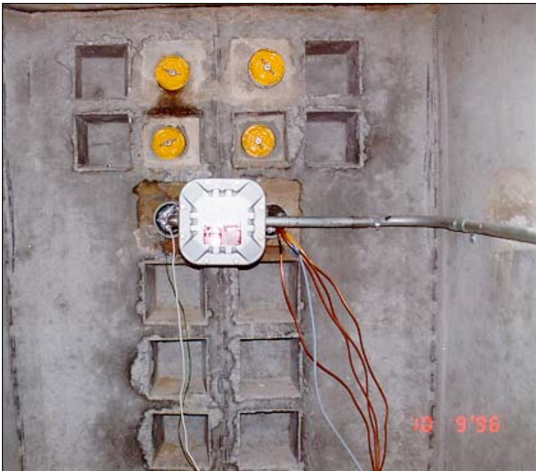
Figure 3-1 Photograph of the East Wall of the M11 Manhole Showing the Feed Tubes Entering the Manhole
