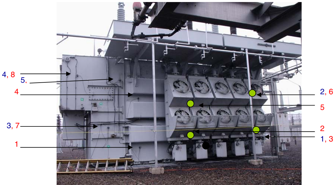
Figure 3-2 Location of acoustic sensors on HV side
