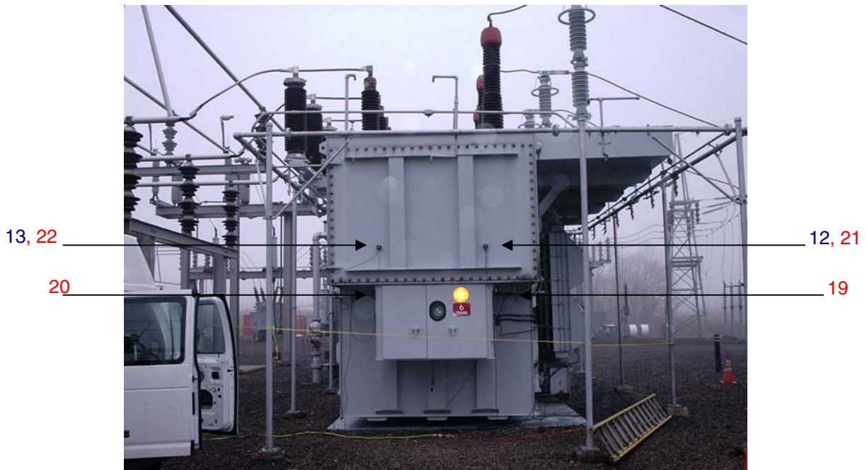
Figure 3-5 Location of acoustic sensors on Load Tap Changer compartment side
