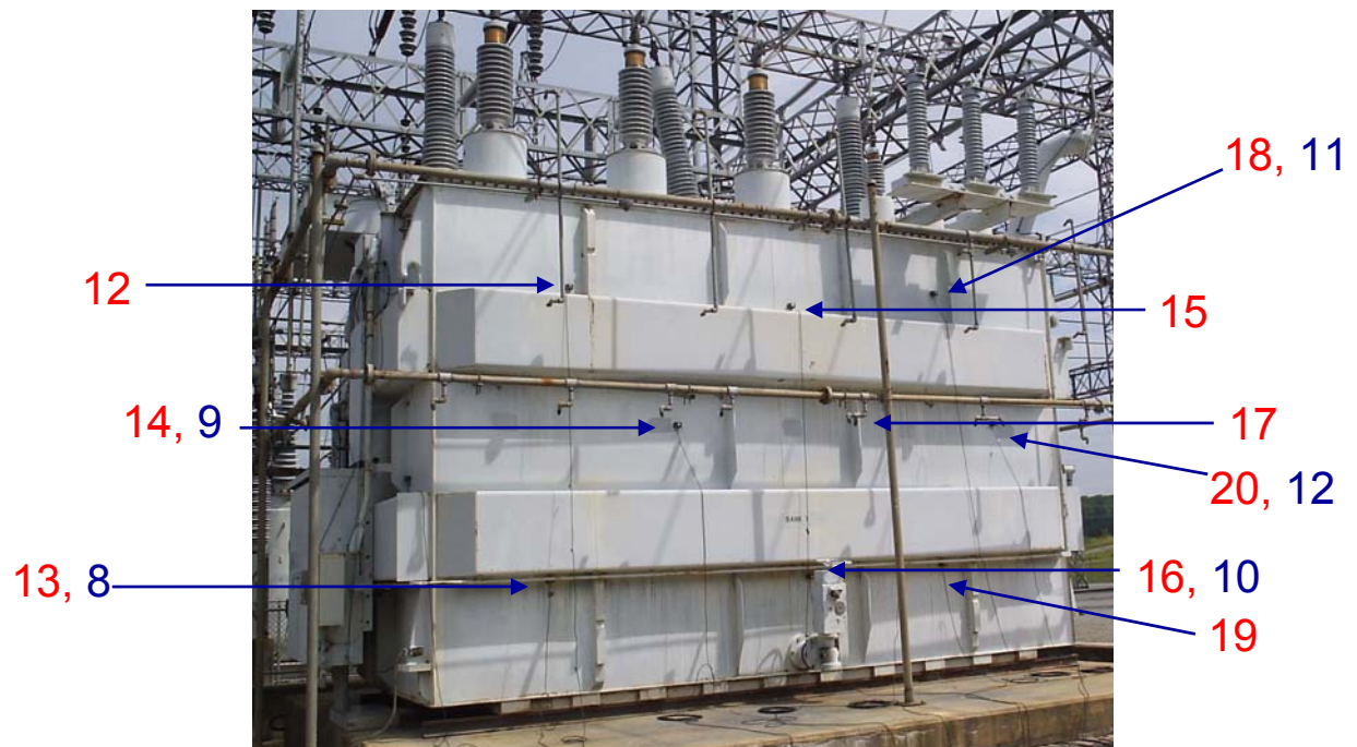
Figure 3-13 Sensor location Low Voltage Side
