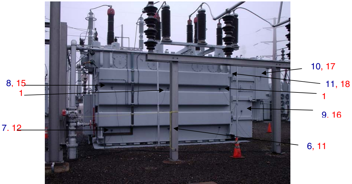
Figure 3-4 Location of acoustic sensors on LV side
