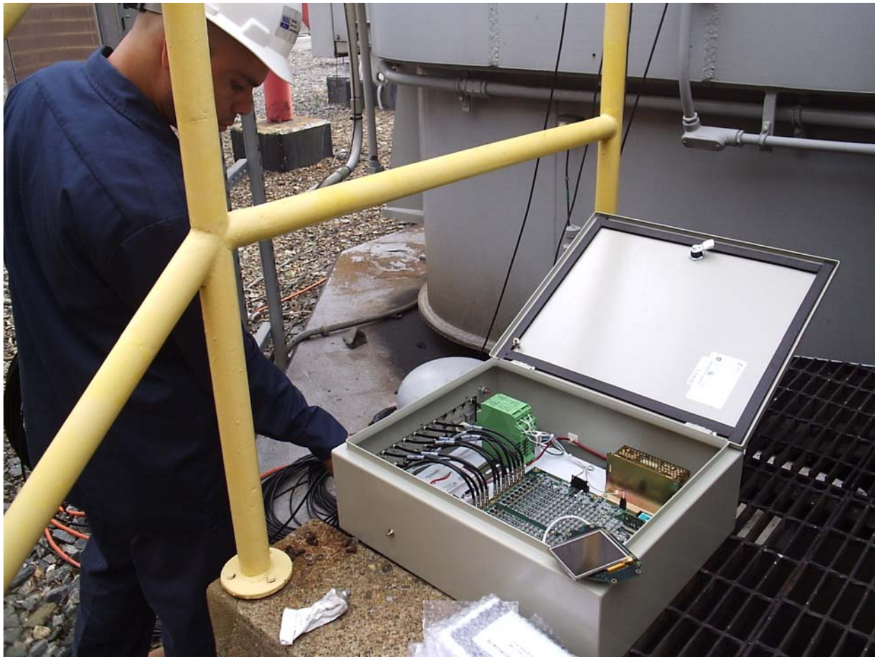
Figure 2-6 Installation on-site of the acoustic sensors and parametric channel
