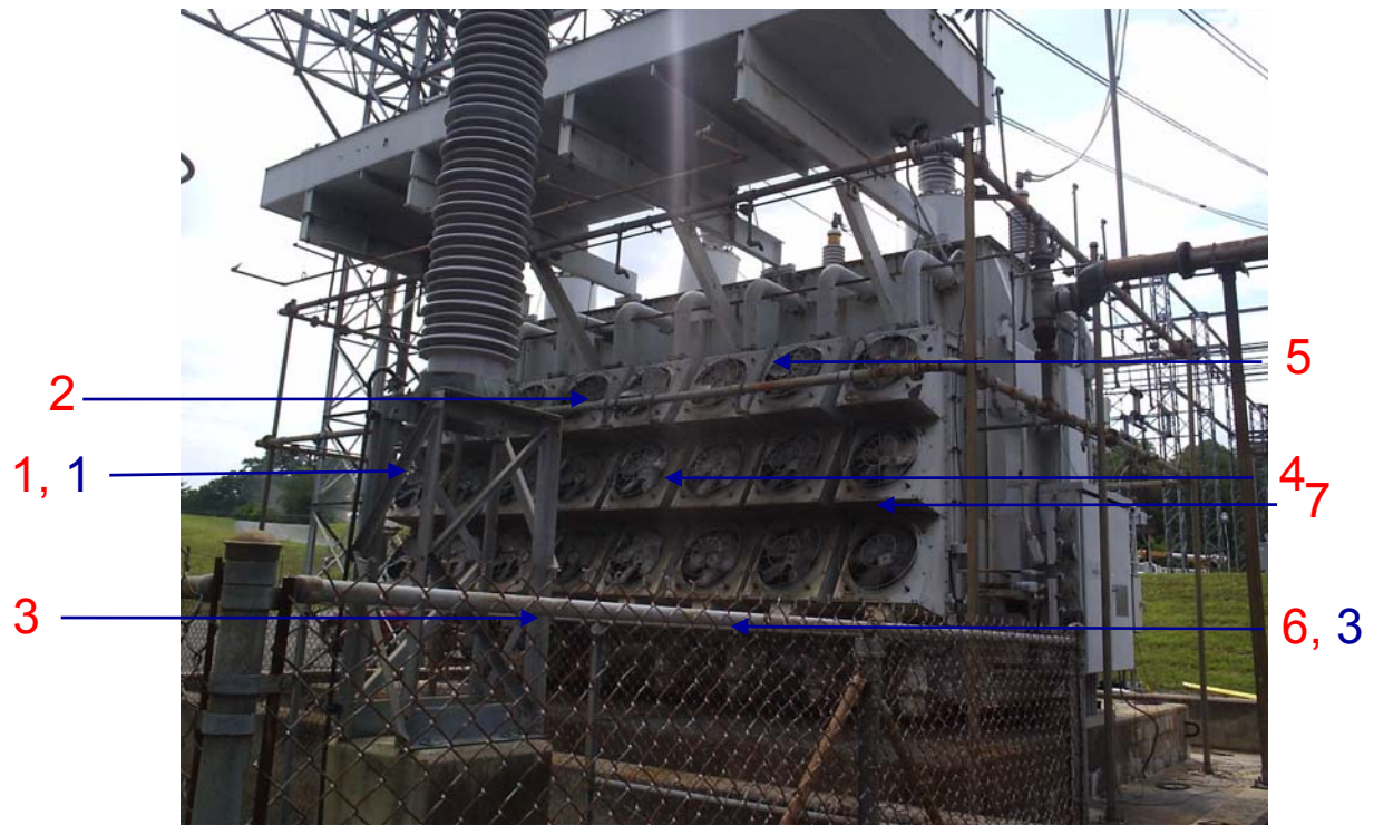
Figure 3-11 Sensor location HV side
