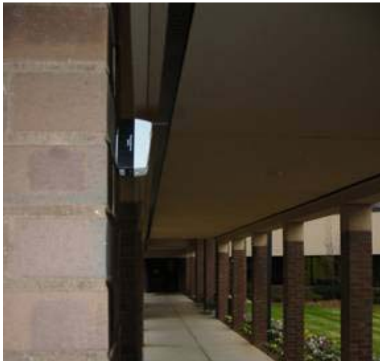
Figure 4-3 A node on a pillar along the secondary path
