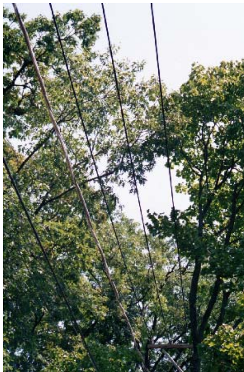
Figure 5-4 Lines With Significant Tree Overhang
