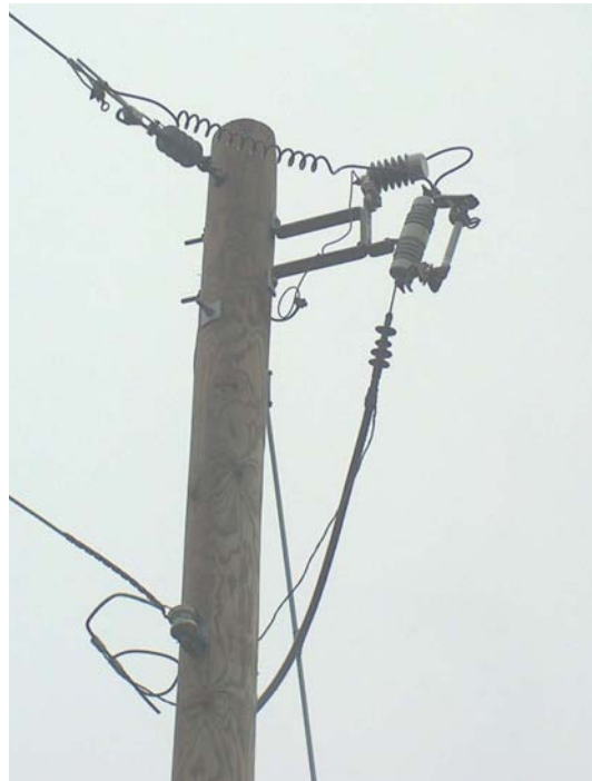
Figure 2-3 Excessive Arrestor Ground Lead Length The phase lead is reasonably short but the arrester ground lead should be bonded directly to the termination.
