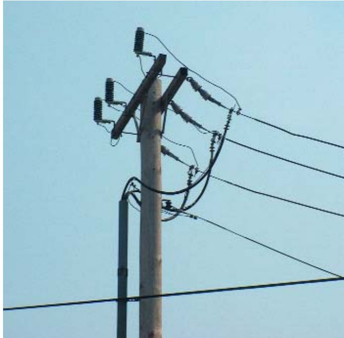
Figure 2-2 Example of Excessive Arrestor Lead Length (both phase and ground leads)
