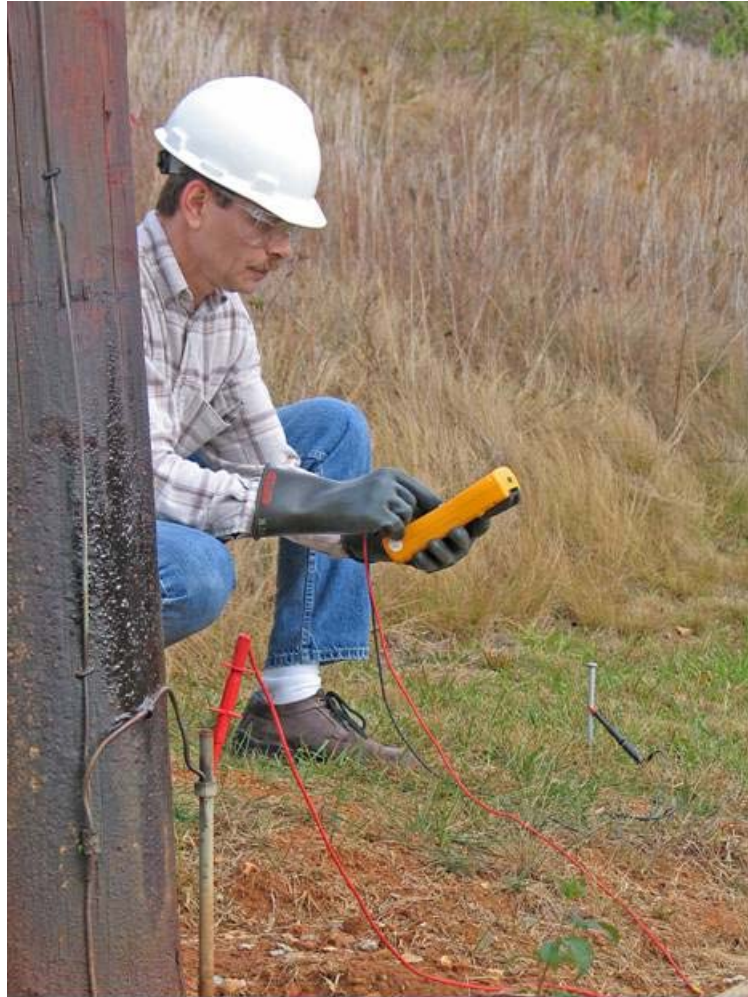
Figure 7-12 Sample Measurements Between a Pole Down Ground and a Reference Ground
