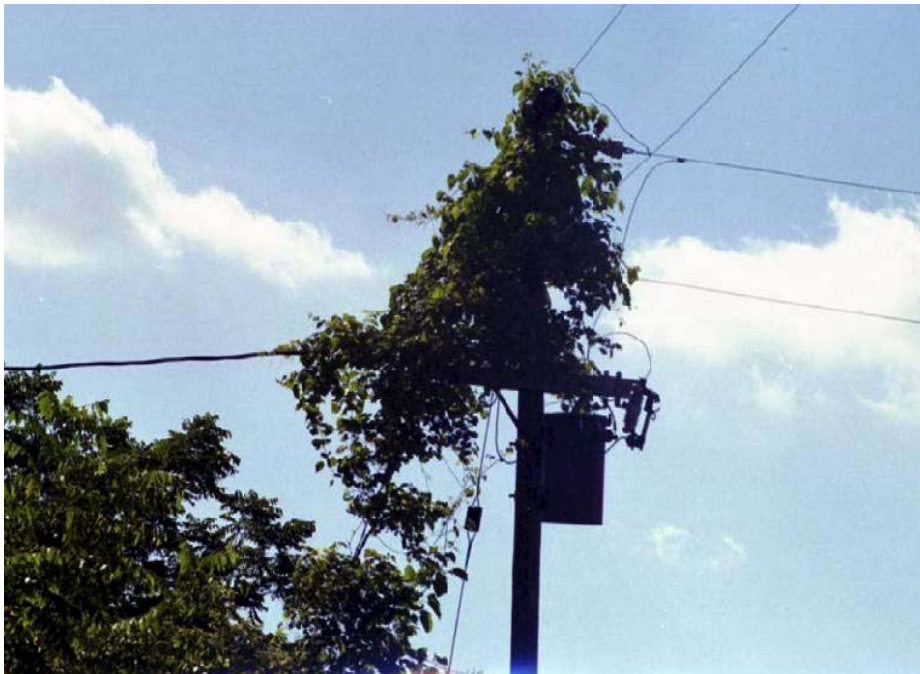
Figure 2-15 Heavy Vine Growth on Pole
