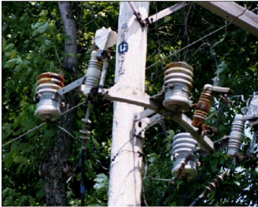
Figure 2-12 Flashed Potheads, Cutouts, and Arresters
