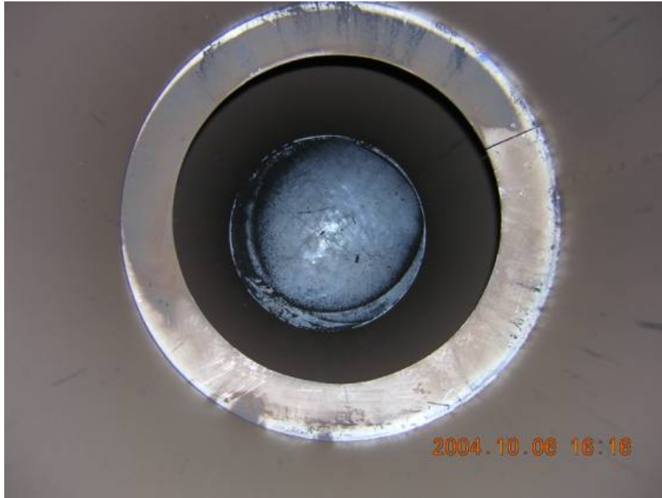
Figure 3-1 Photo of a concentric orifice installed just upstream of a bend
