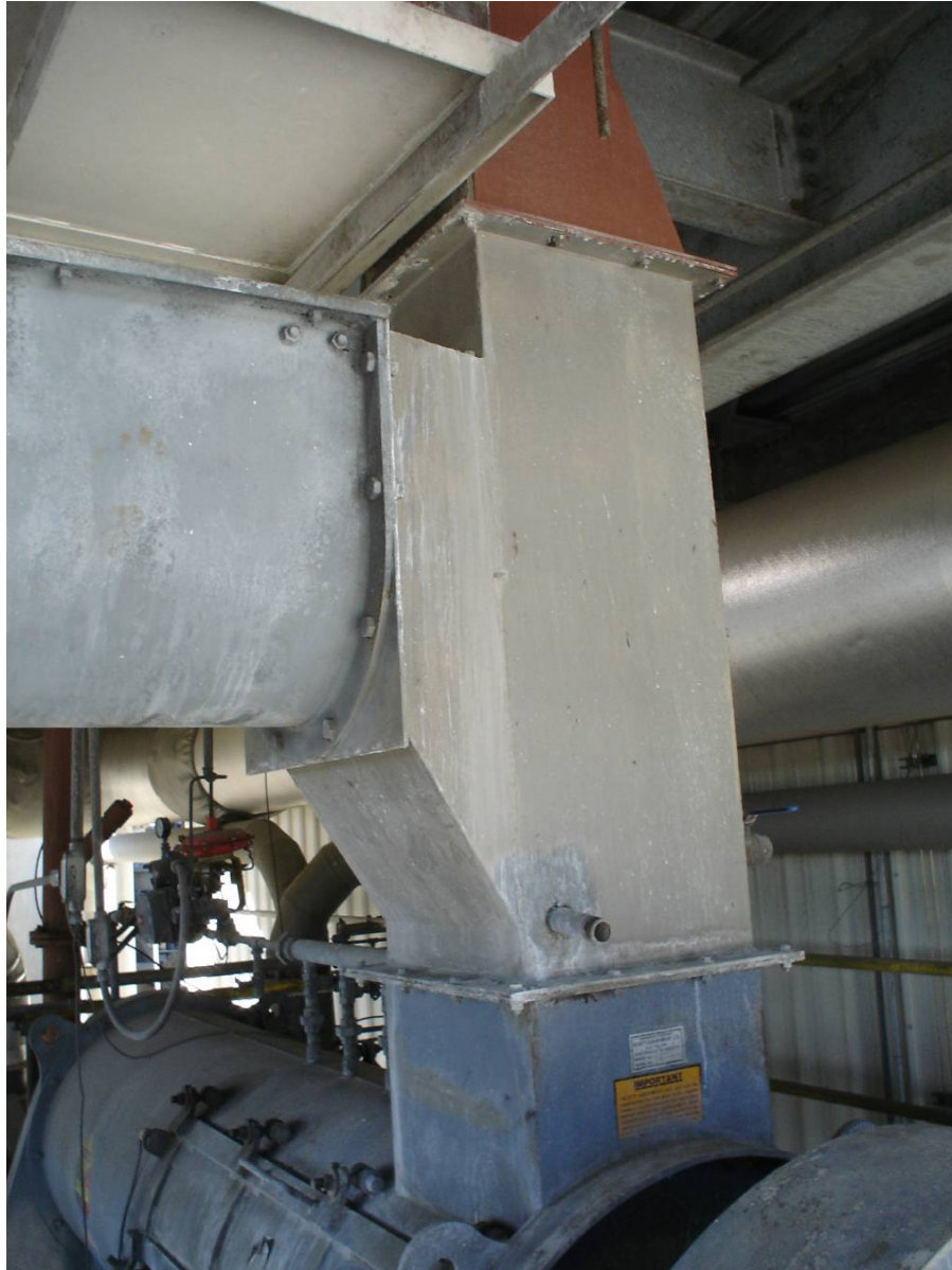
Figure 3-3 Alkali Metering and Addition to Fly Ash above High Intensity Mixer
