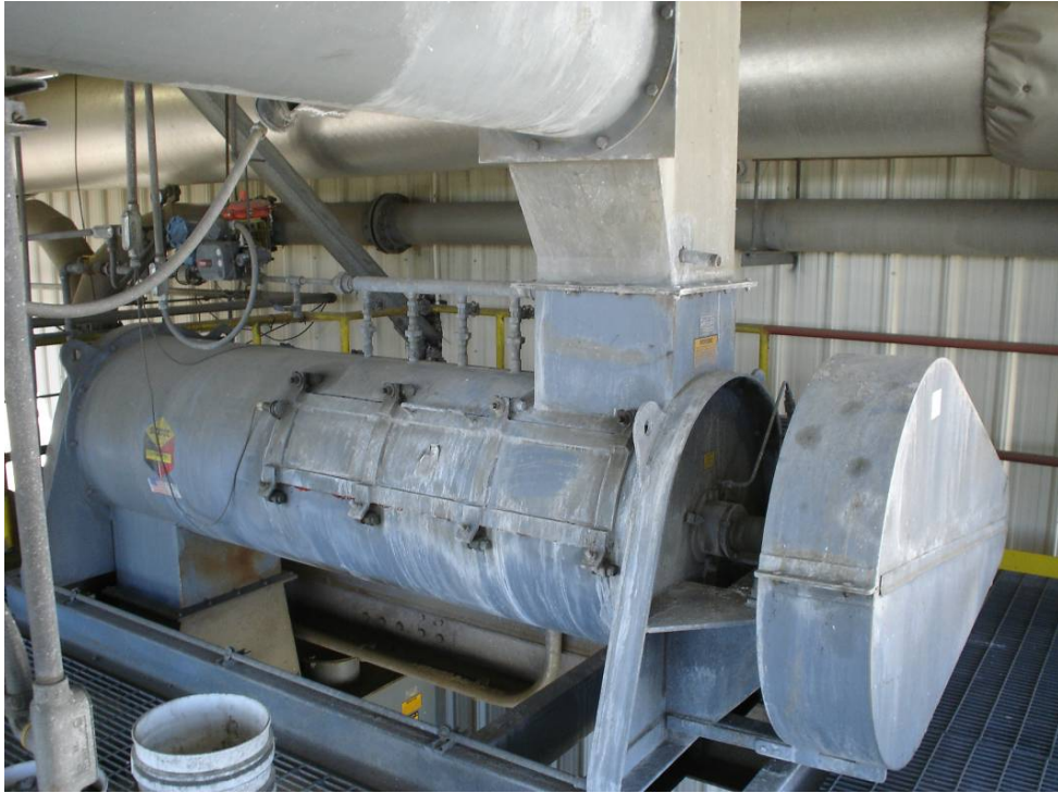
Figure 3-4 High-Intensity Rotary Mixer
