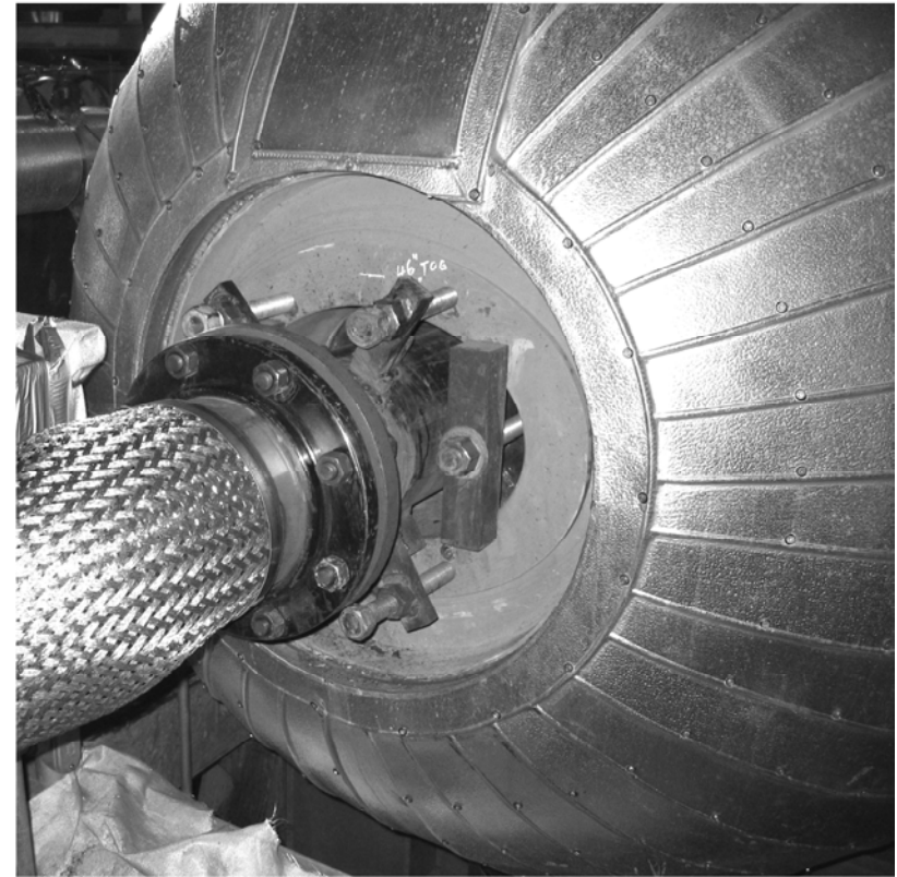
Figure 2-2 Case Study 1: Steam Drum Manway Connection for Temporary Chemical Cleaning Piping
