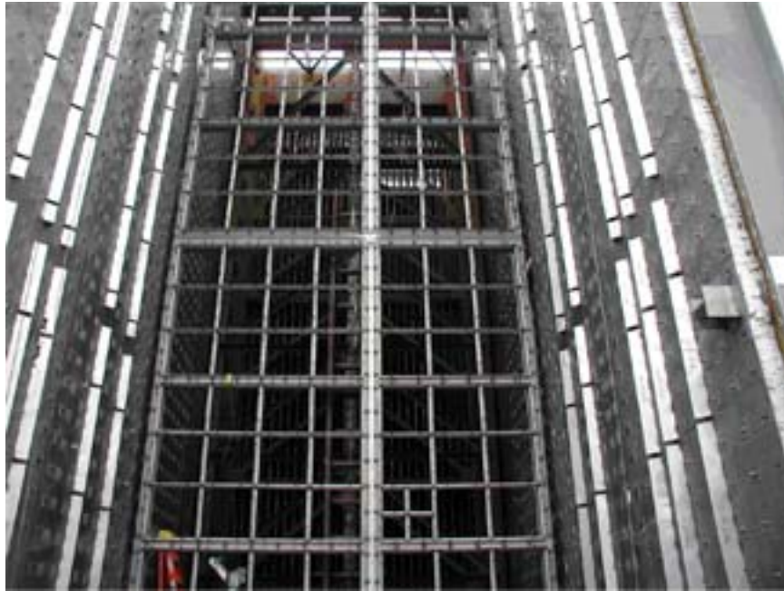
Figure 2-1 Photograph of a Partially Finished HRSG Assembly
