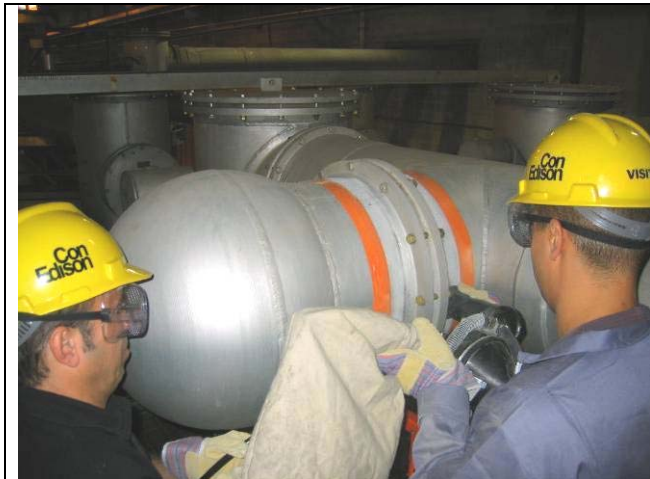
Step 1: Surface Preparation
