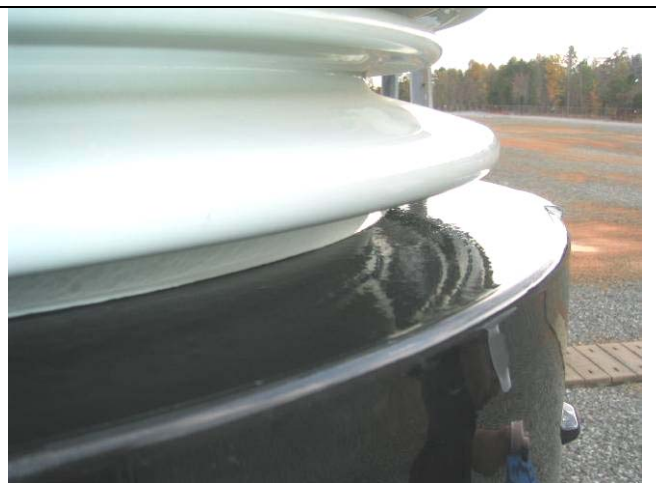
Step 4: Application of the sealing resin
