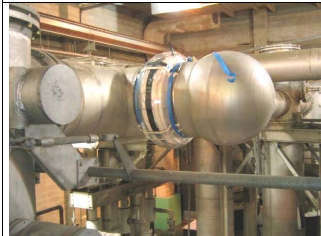
Step 3: Application of the outer rigid shell
