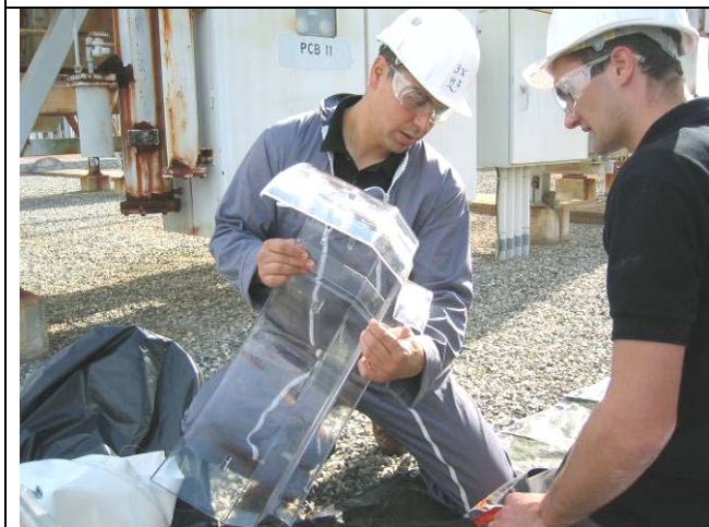
Step 3: Application of the outer rigid shell
