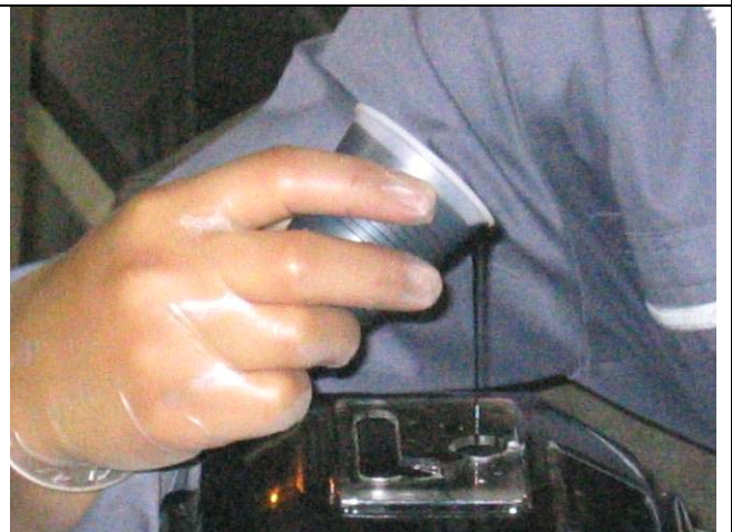
Step 4: Application of the sealing resin
