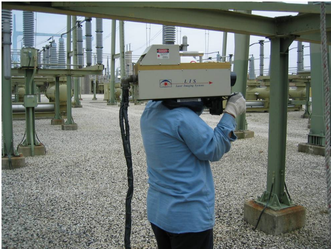
Figure 1 - Application of the GasVue camera for location of the SF 6 leaks
