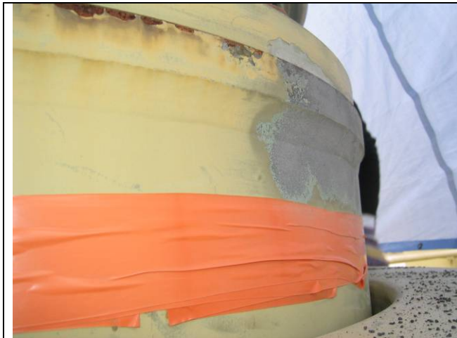
Step 1: Surface Preparation
