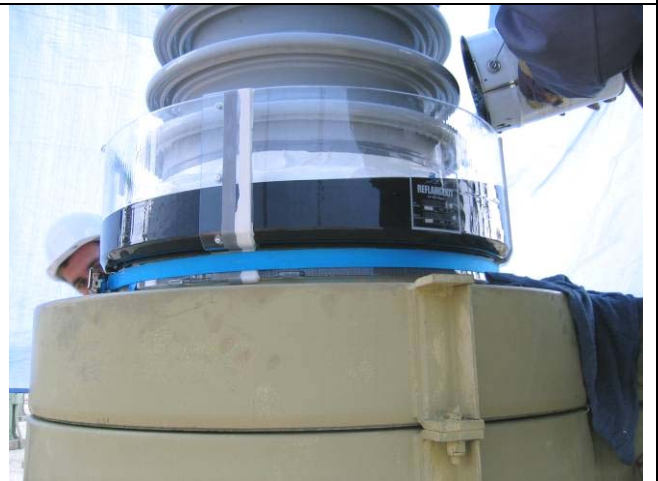
Step 4: Application of the sealing resin
