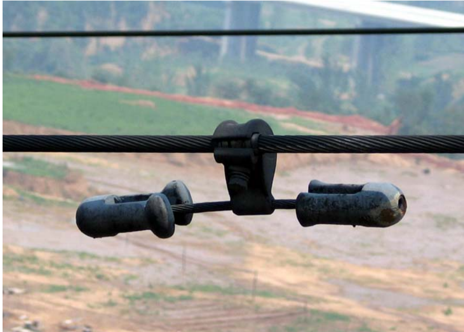
Figure A-12 Evidence of a Sparkover (Burn Mark) on Conductor Hardware
