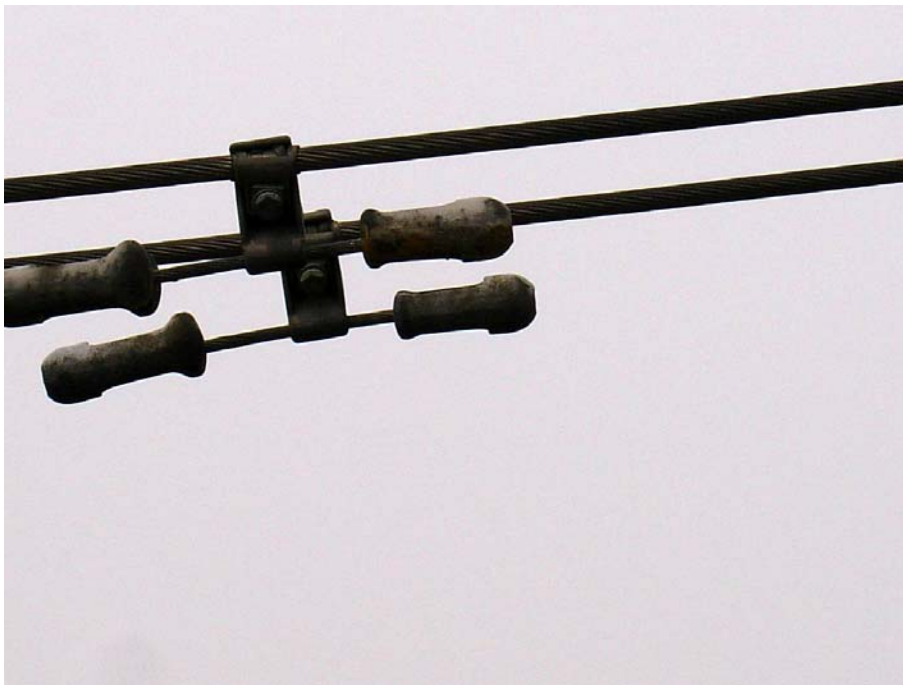
Figure A-11 Evidence of a Sparkover (Burn Mark) on Conductor Hardware
