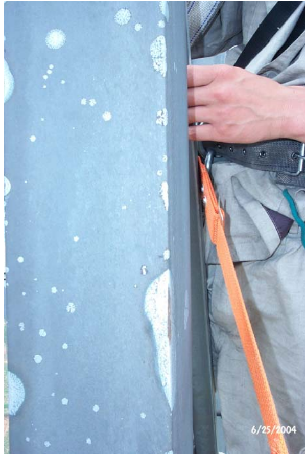
Figure A-6 Evidence of a Sparkover (Burn Mark) on a Steel Lattice Member
