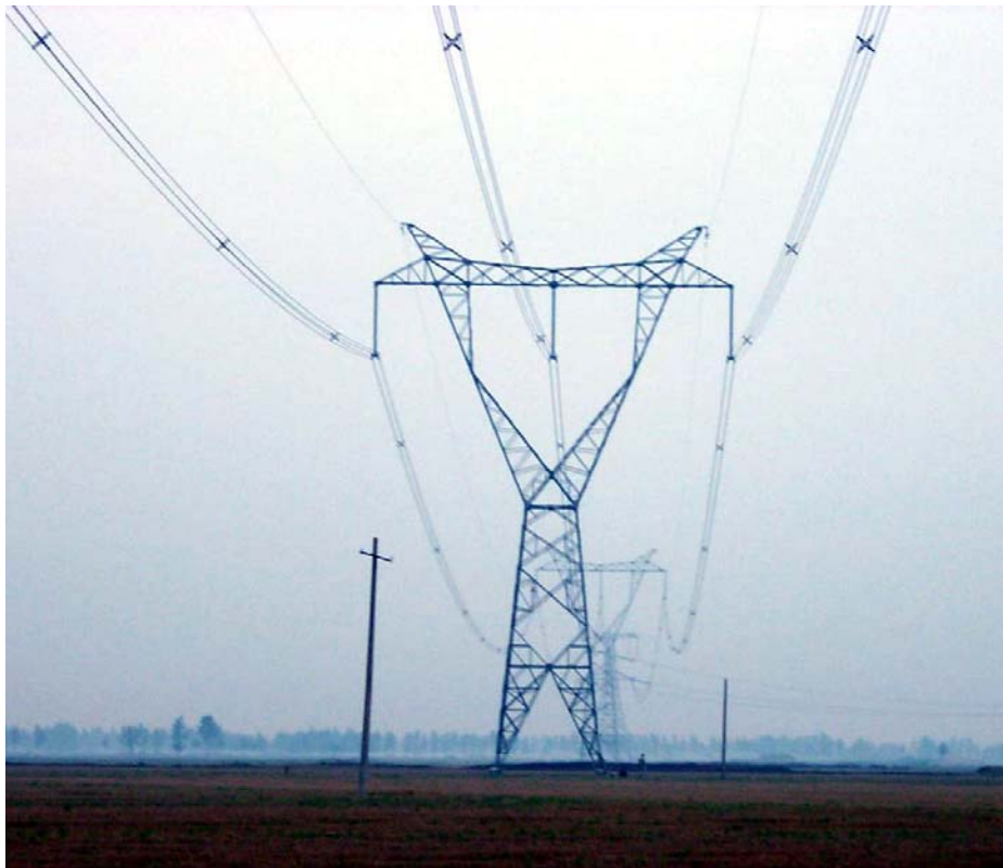
Figure 1-1 Typical Henan Tangent Single-Circuit 500-kV Steel Lattice Structures
