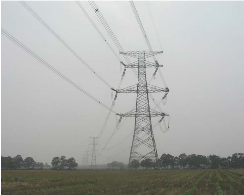
Figure 1-2 Typical Henan Dead-End and Tangent Double-Circuit 500-kV Steel Lattice Structures (Courtesy of Henan Power)
