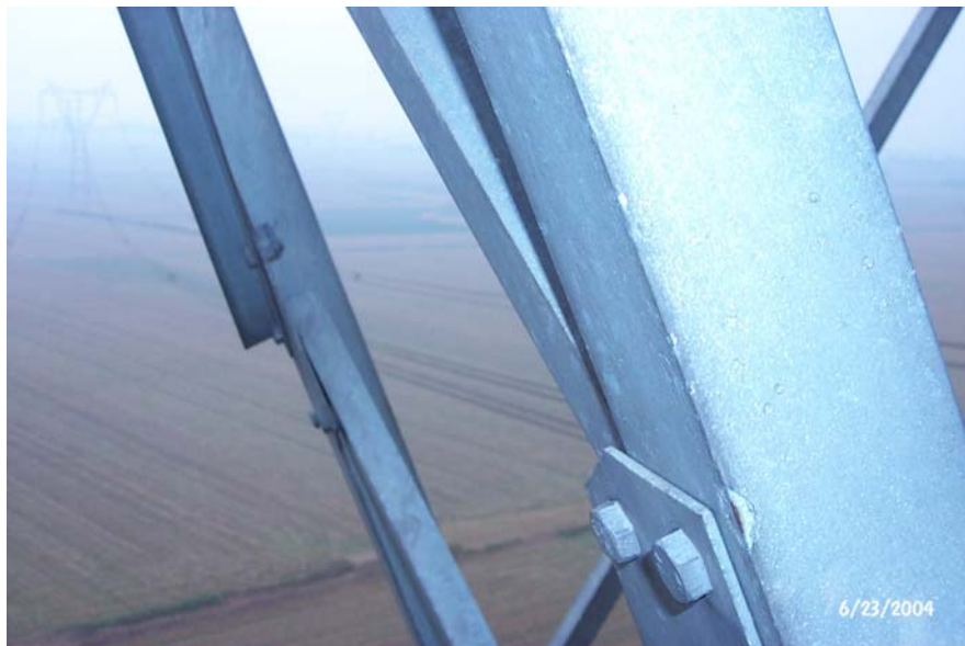
Figure A-1 Evidence of a Sparkover (Burn Mark) on a Steel Lattice Member
