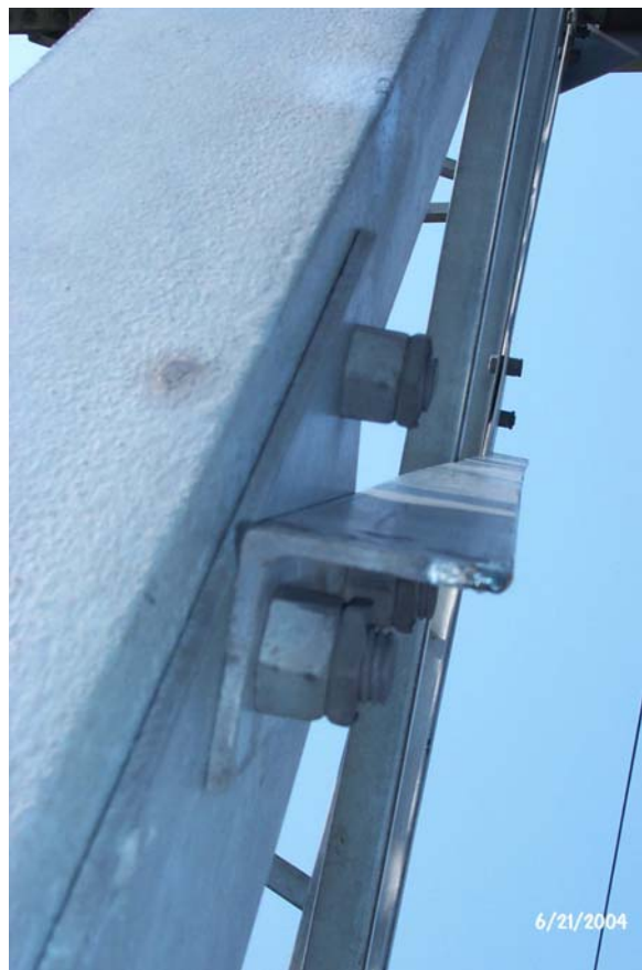
Figure A-5 Evidence of a Sparkover (Burn Mark) on a Steel Lattice Member
