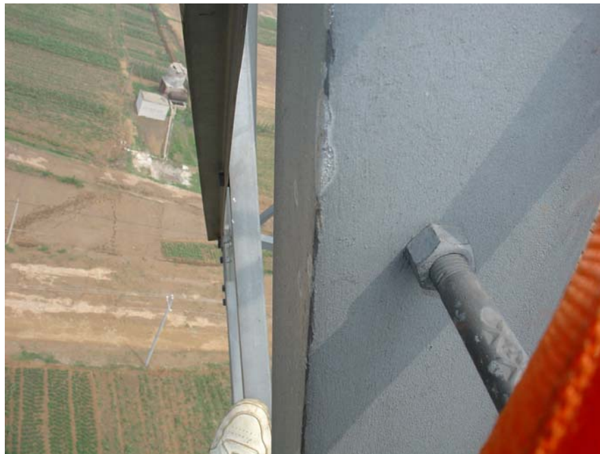
Figure A-3 Evidence of a Sparkover (Burn Mark) on a Steel Lattice Member
