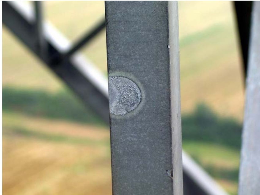
Figure 1-3 Evidence of a Sparkover (Burn Mark) on a Steel Lattice Member
