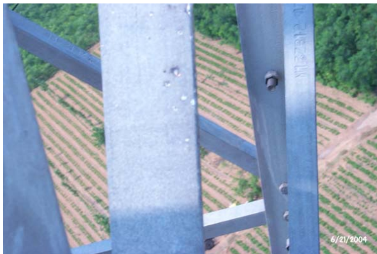
Figure A-7 Evidence of a Sparkover (Burn Mark) on a Steel Lattice Member
