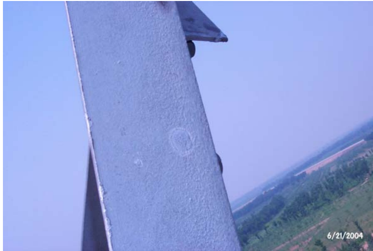
Figure A-4 Evidence of a Sparkover (Burn Mark) on a Steel Lattice Member
