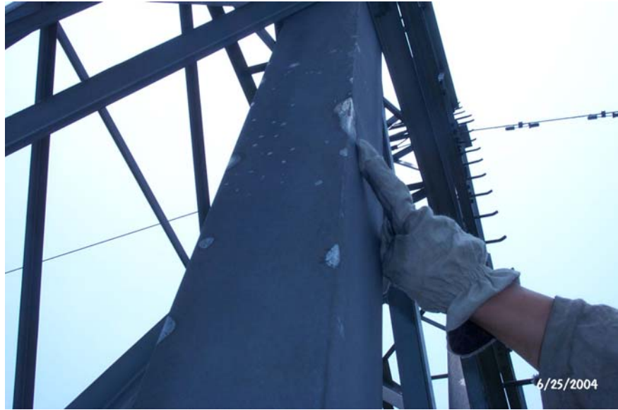
Figure A-2 Evidence of a Sparkover (Burn Mark) on a Steel Lattice Member
