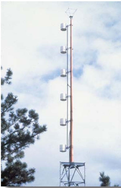
Figure 5. FM radio broadcast antennas. Photo reprinted with permission from Richard Tell Associates, Inc.
