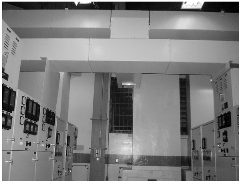
Figure 3-6 Diablo Canyon Bus Duct Repair (external view)
