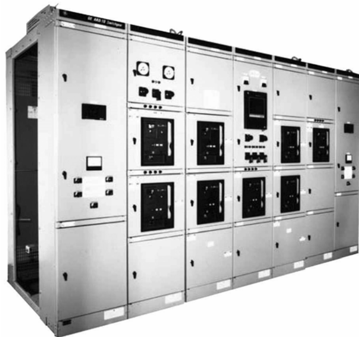
Figure 2-2 General Electric AKD-10 Low-Voltage Switchgear
