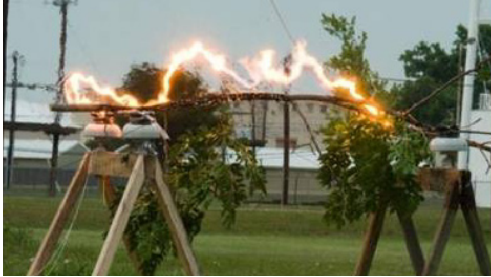
Figure 4-4 Arcing Rising With Hot Plasma and Forming Jacob's Ladder
