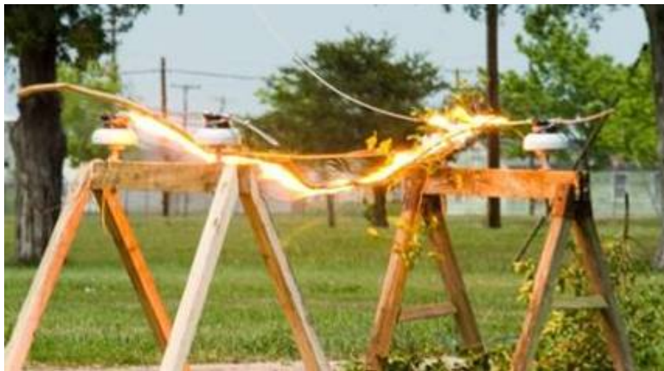
Figure 4-3 Arcing and Burning of Tree Limb Bridging Two Conductors
