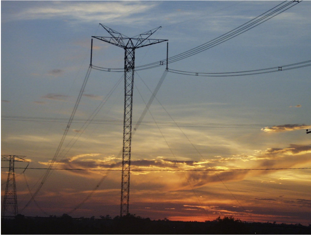
Figure 5-3 FURNAS \pm 600 kV HVDC Line
