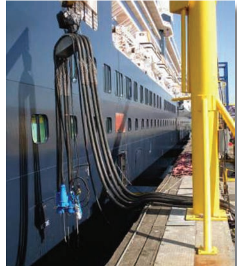
Figure 3. Shore Power Cables (photo courtesy of Mike Watts, Cochran Electric)
