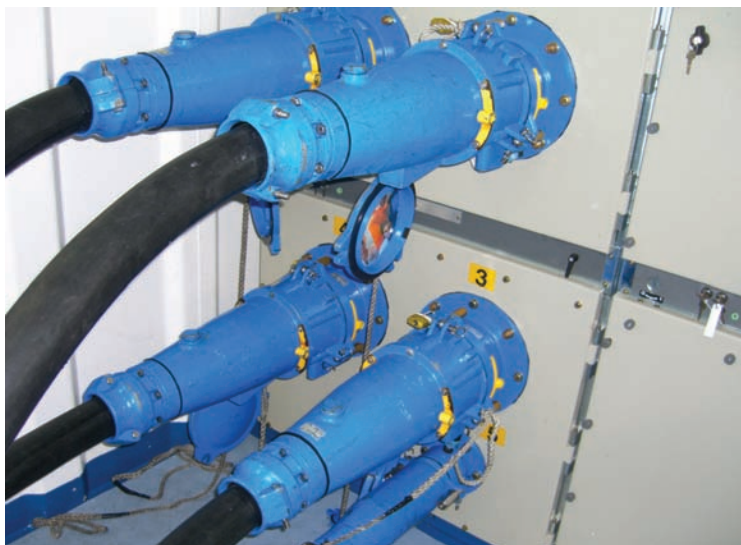
Figure 4. Cable Connection on Board Holland America Ship (photo courtesy of Brian Sisco, Southern California Edison)
