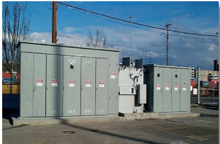
Figure 2. Shore Power Transformer and Metering Equipment at Port of Seattle (photo courtesy of Mike Watts, Cochran Electric)
