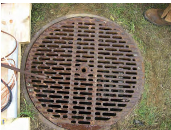
Figure 1-4 Steel Cover with Unclogged Slots
