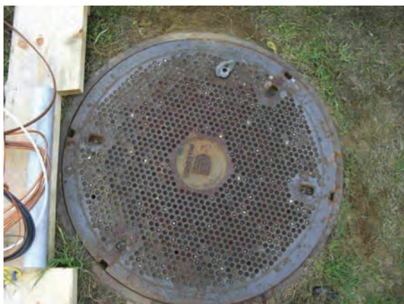
Figure 1-2 Steel Cover with Clogged Vent Holes
