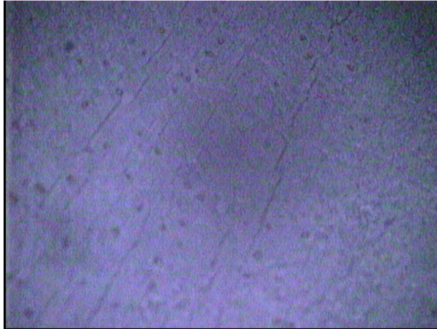
Figure 5-6 Multiple Longitudinal Cracks Found in an Economizer Tube (This type of cracking is indicative of thermal fatigue from hot/cool or wet/dry cycles.)
