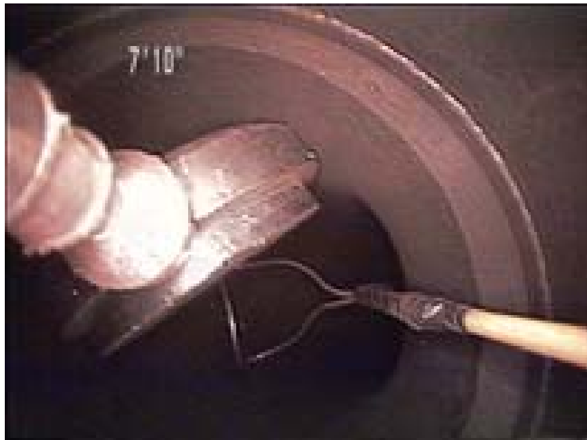
Figure 11-1 Location and Positioning of a Retrieval Tool for a Blanking Plate Using RVI to Assist the Operation
