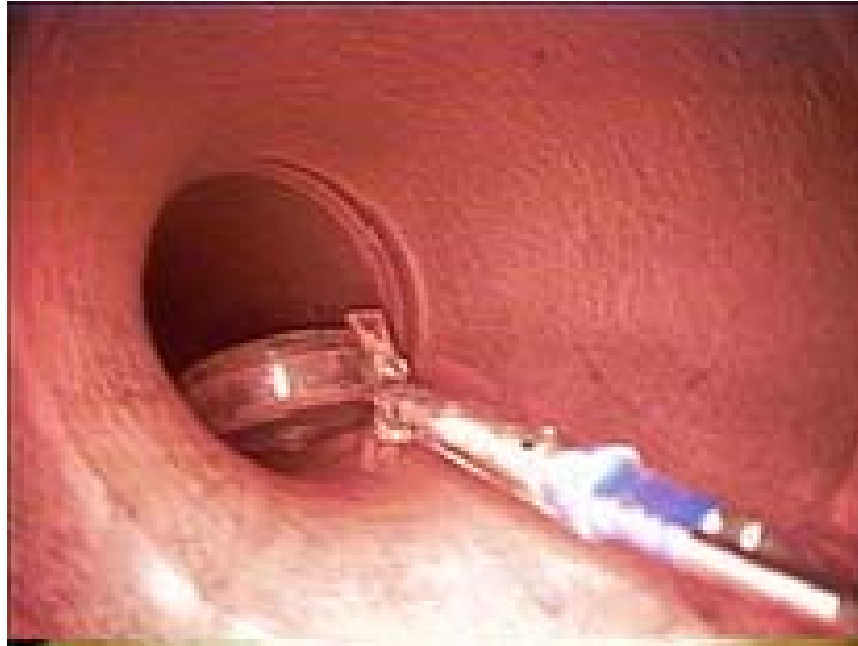
Figure 11-2 Removal of a Blanking Plate with a Snare Using RVI
