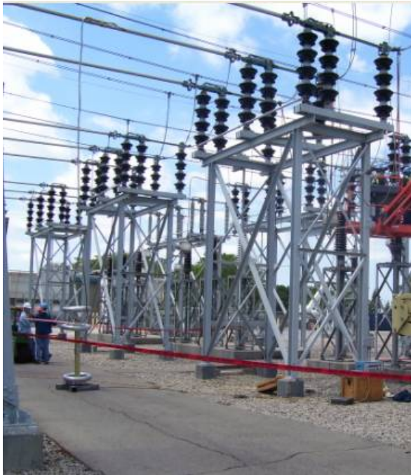
Figure 4-24 Dissipation factor measurement equipment connected to NYPA high voltage bus
