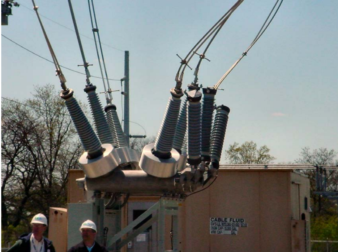
Figure 3-7 SF 6 Circuit Breaker
