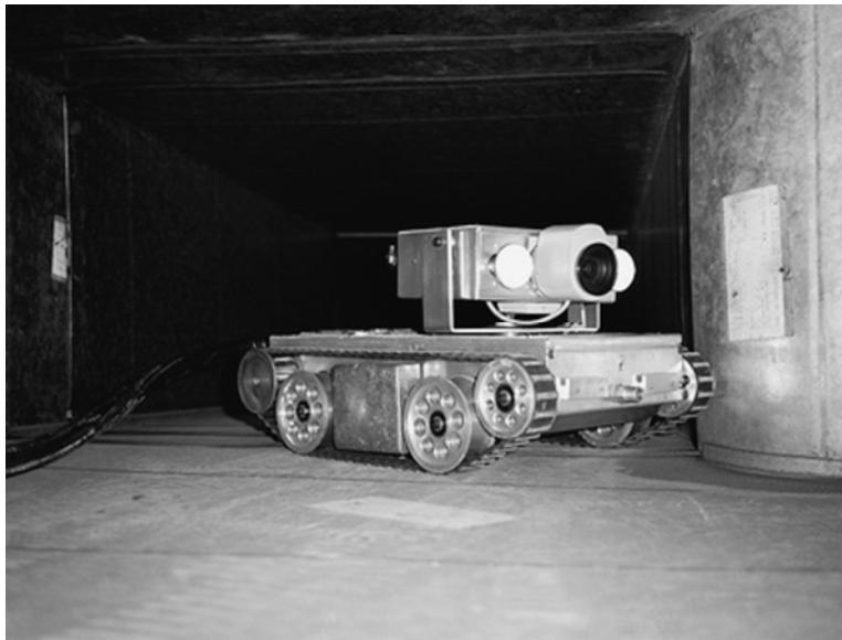
Figure 11-8 Robotic Walkers Are Ideal for Performing and Recording Visual Inspections in Isophase Buses with Limited-Sized Inspection Covers
