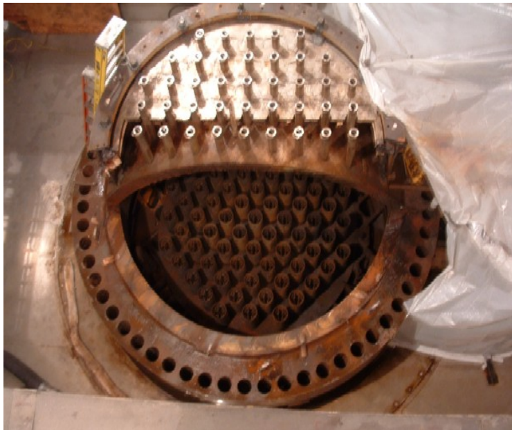
Figure 7-1 Reactor Head With First Piece Removed
