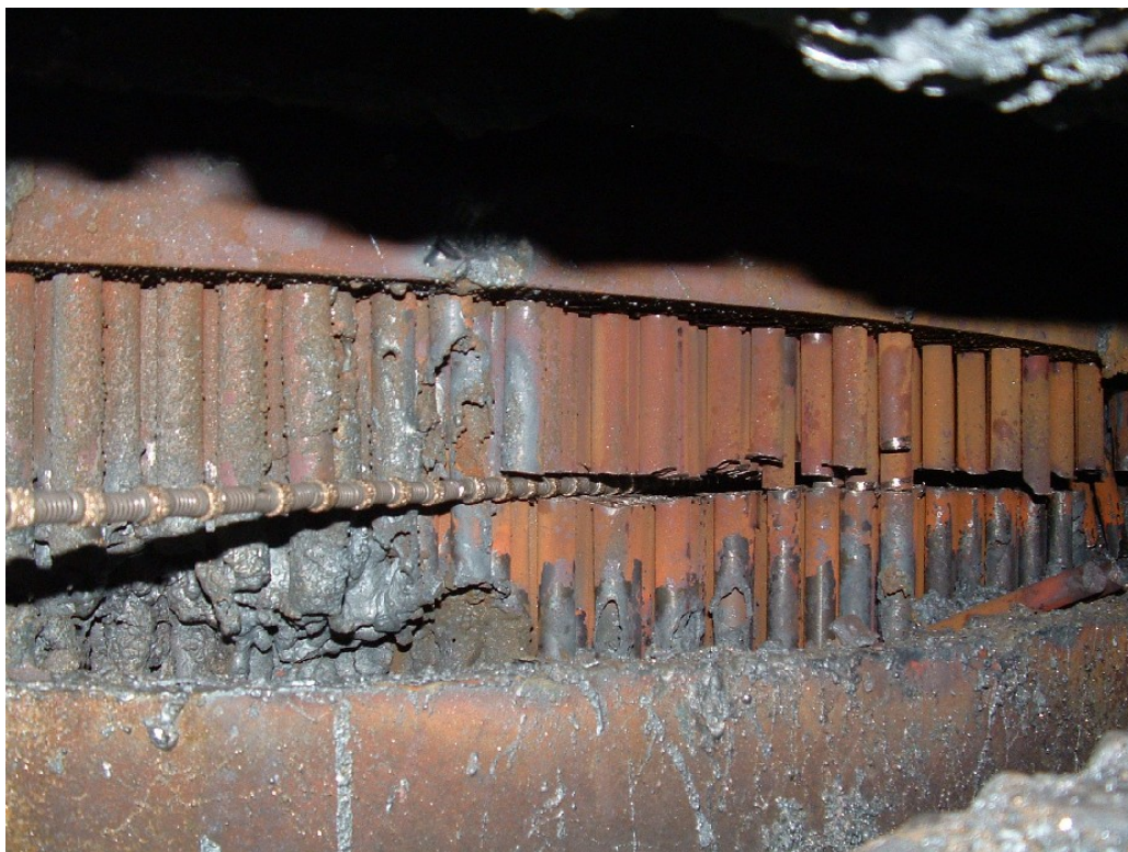
Figure 7-2 Diamond Wire Saw Cutting Tubes Through Window in OTSG Shell
