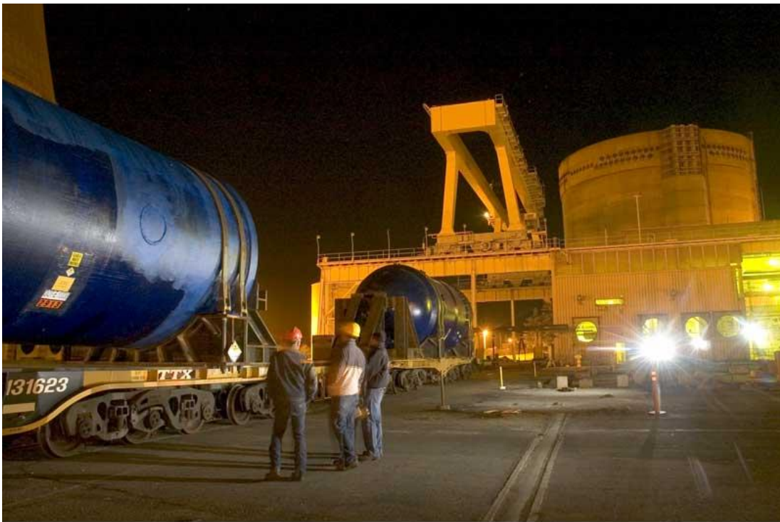
Figure 7-4 Steam Generator Sections Leaving Rancho Seco
