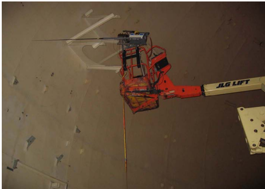
Figure 8-1 Final Status Survey of the Rancho Seco Containment Dome With ISOCS
