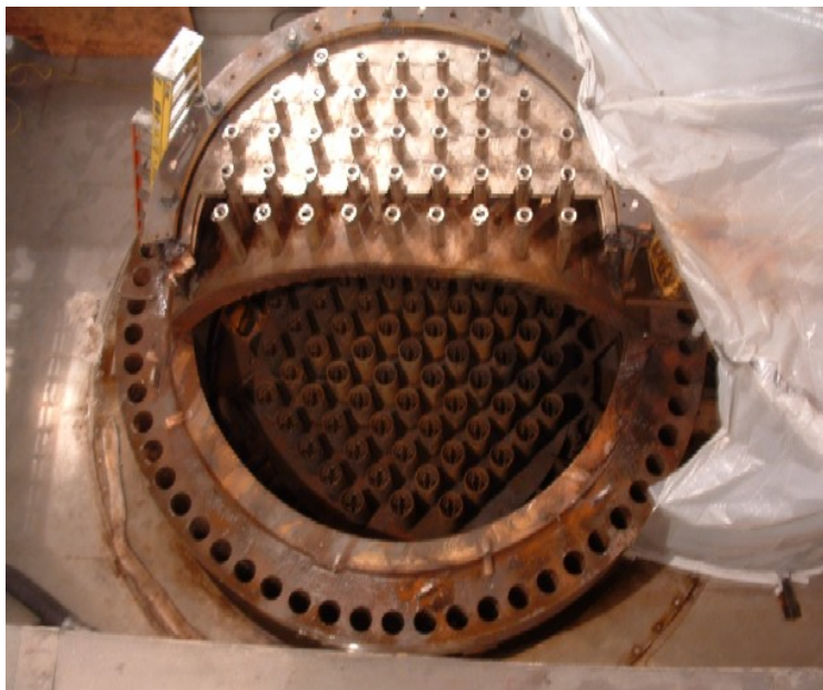
Figure 7-1 Reactor Head With First Piece Removed
