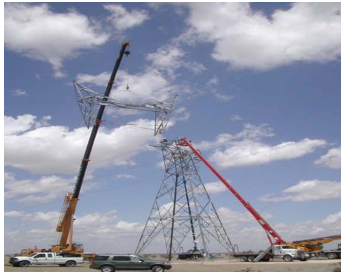
Figure 2-1 Crews Prepare to Attach the Bridge of a 500 kV Steel Lattice Tower
