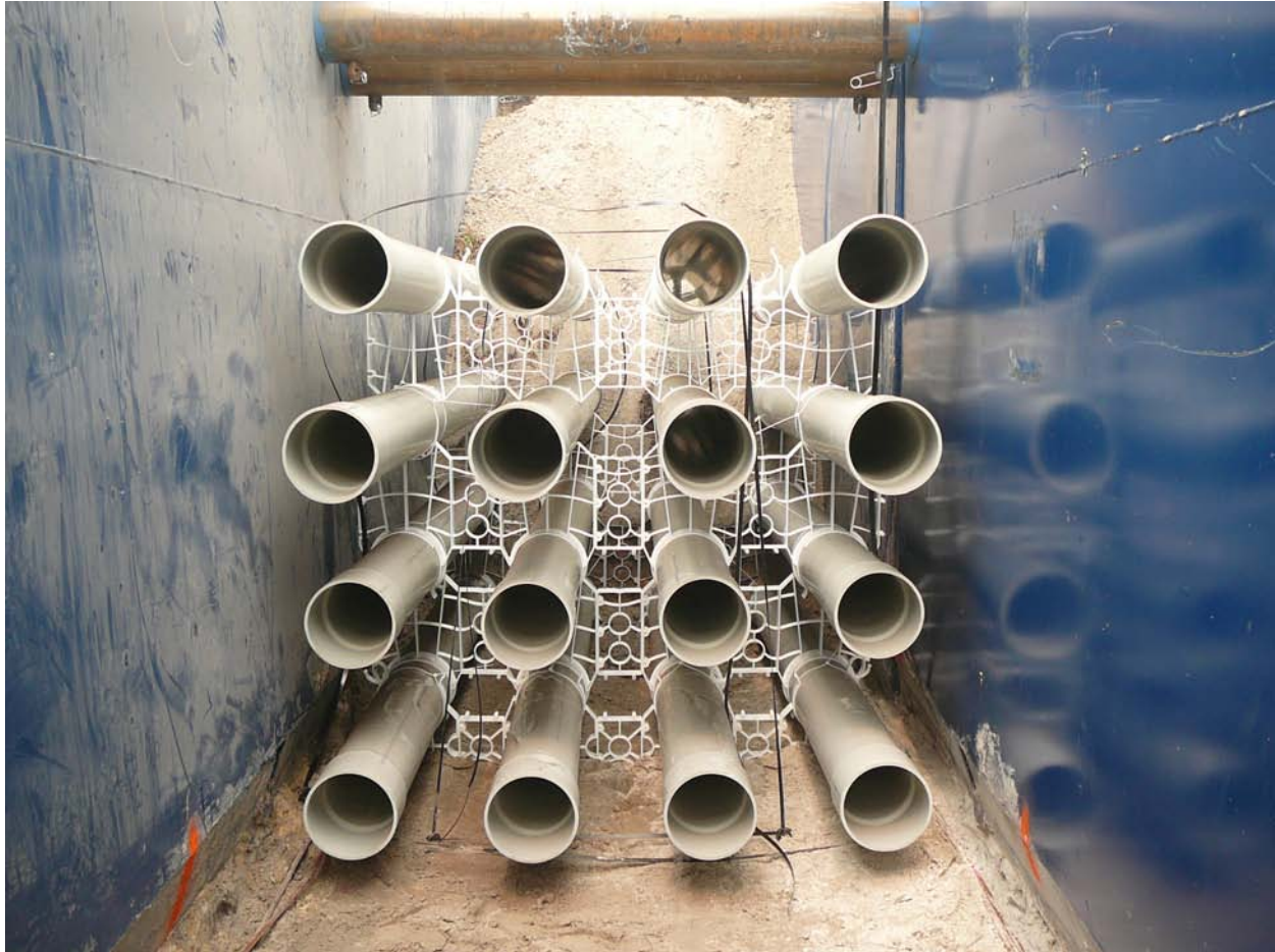
Figure 2-6 Conduits Set into an Open Cut Trench
