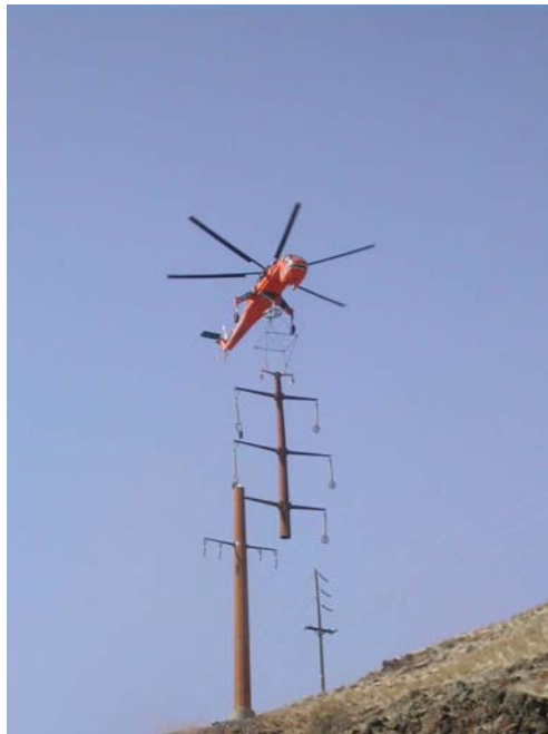
Figure 2-4 A Helicopter Prepares to Set the Top Half of a 345 kV Single Pole Structure
