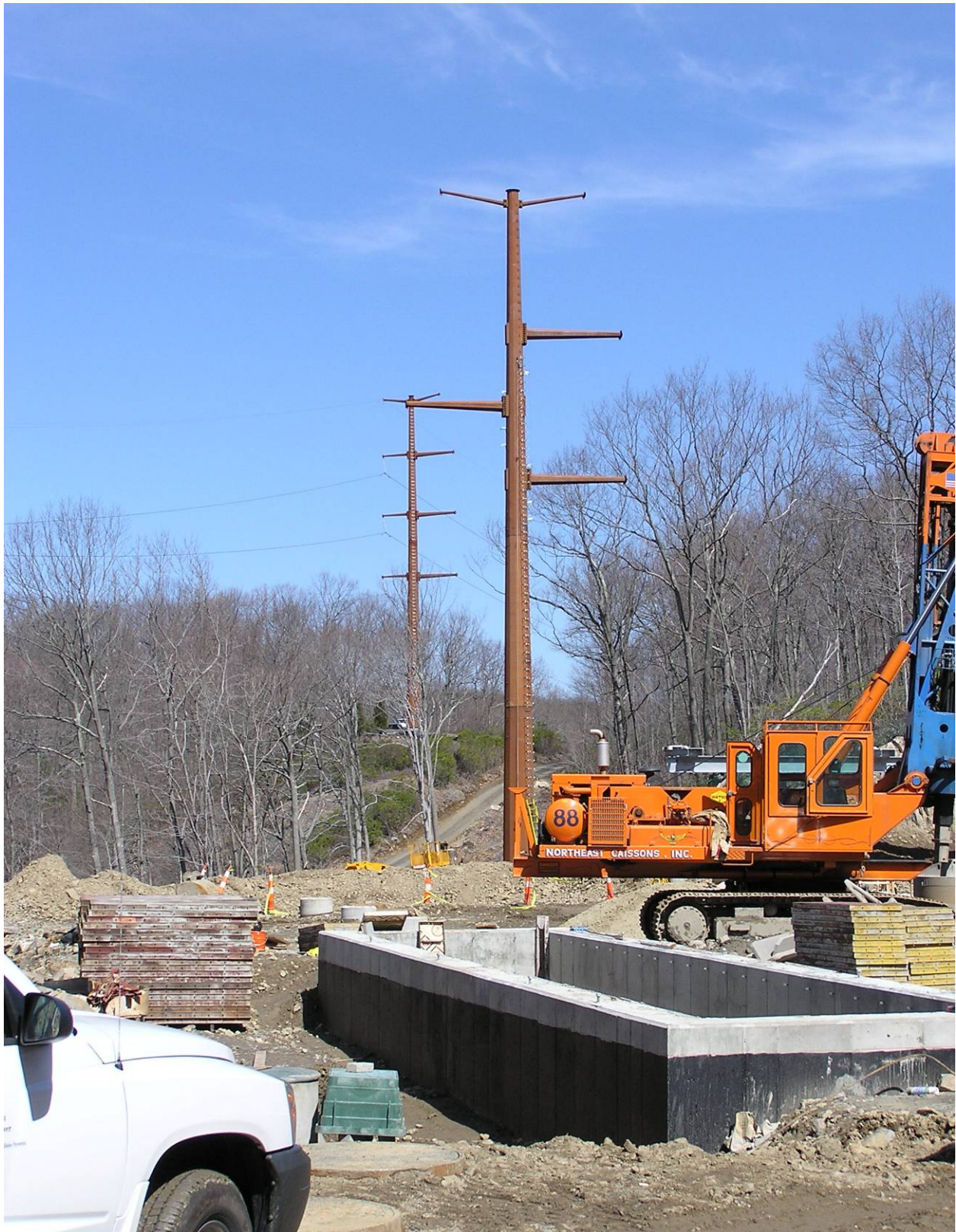
Figure 6-1 Concrete Vault Being Prepared to Transition a 345 kV Overhead Line to Underground
