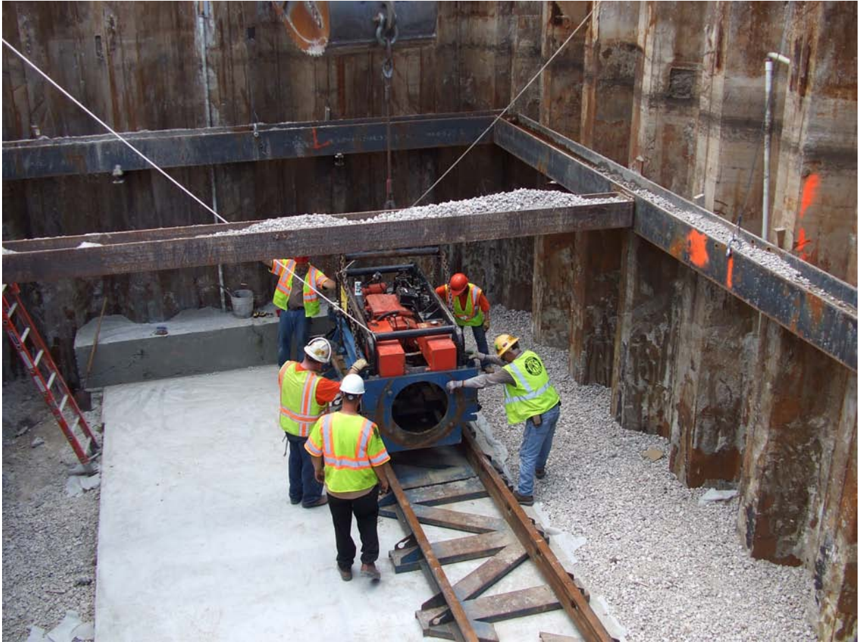
Figure 2-10 Workers Implement Jack & Bore Technique
