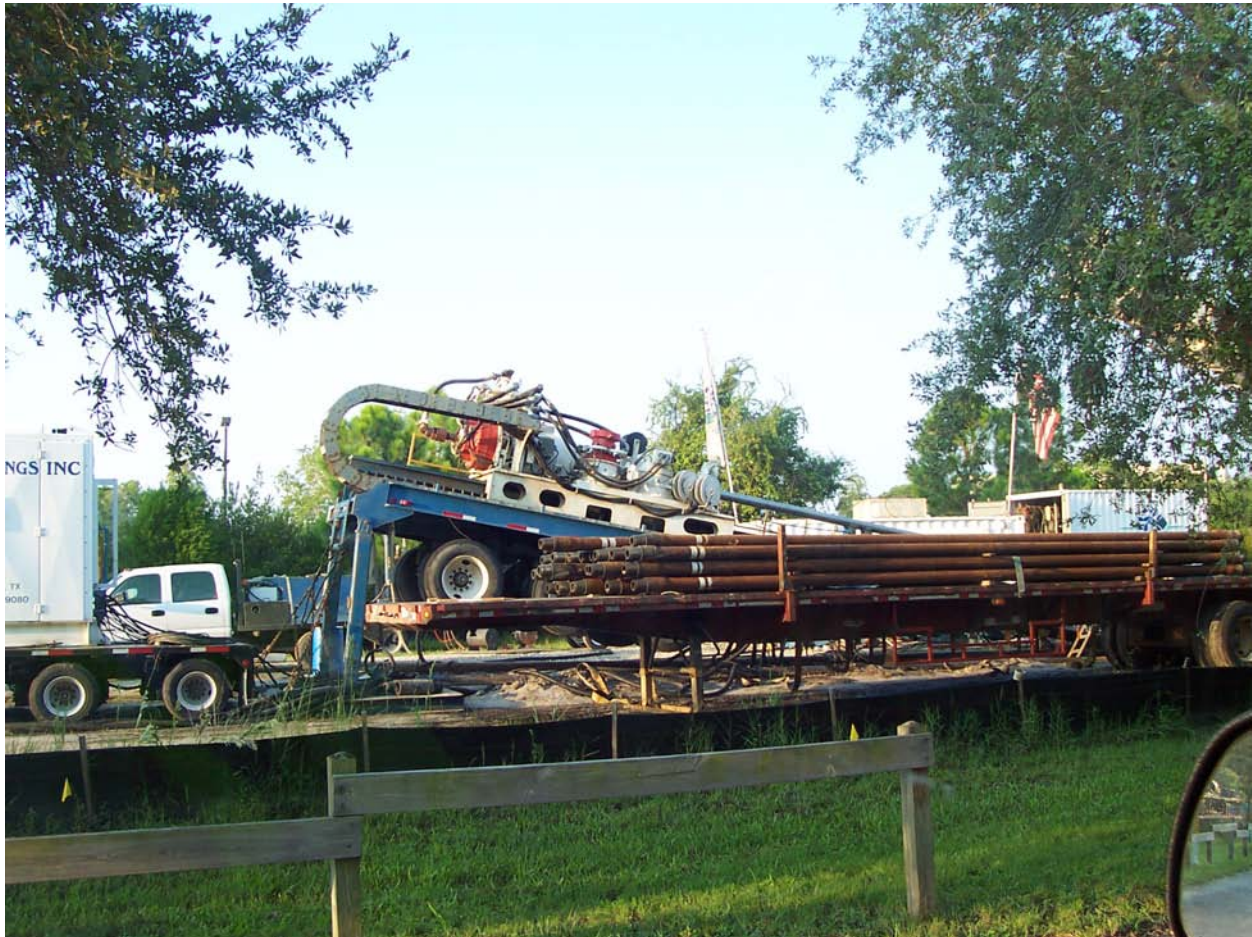
Figure 2-8 Horizontal Directional Drill Pipes
