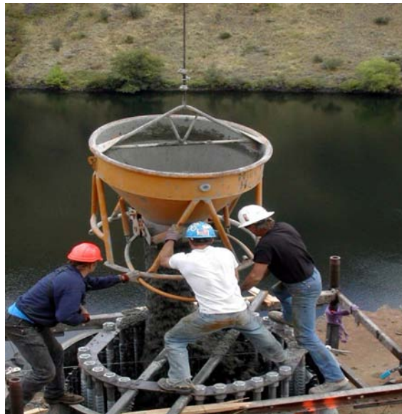
Figure 2-3 Crews Filling a Caisson Foundation for a 230 kV Steel Pole River Crossing
