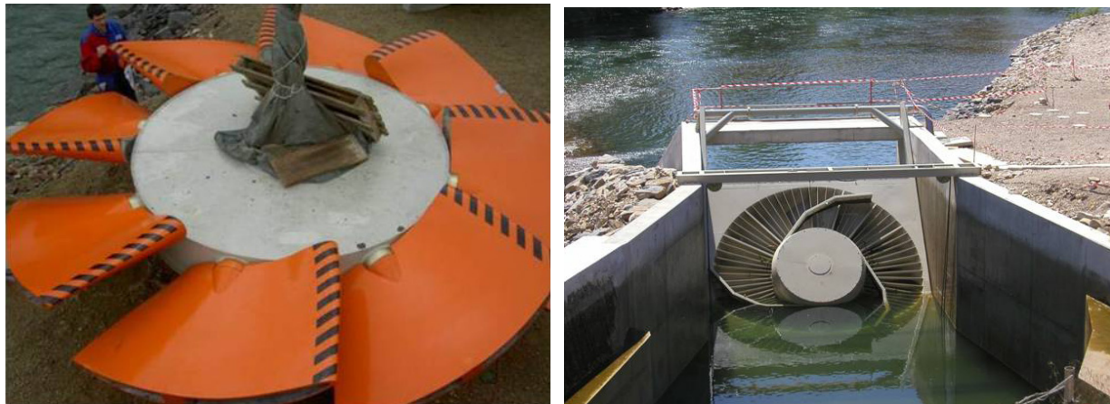
Figure 25-10 Very Low Head (VLH) Turbine Runner (Left Photo) and Full Unit Installed at a Demonstration Site in Millau, France (Right Photo) (Leclerc 2008)
