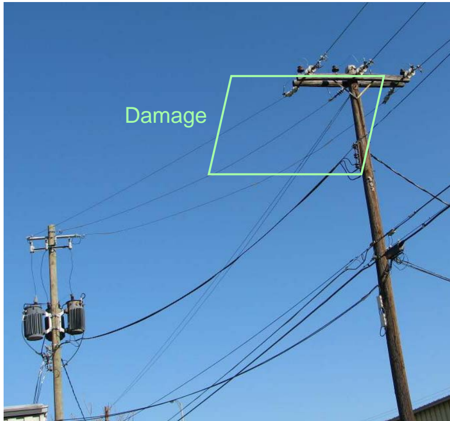
Figure 3-22 Photograph of Line Construction in Area of Wind-Induced Conductor Slap
