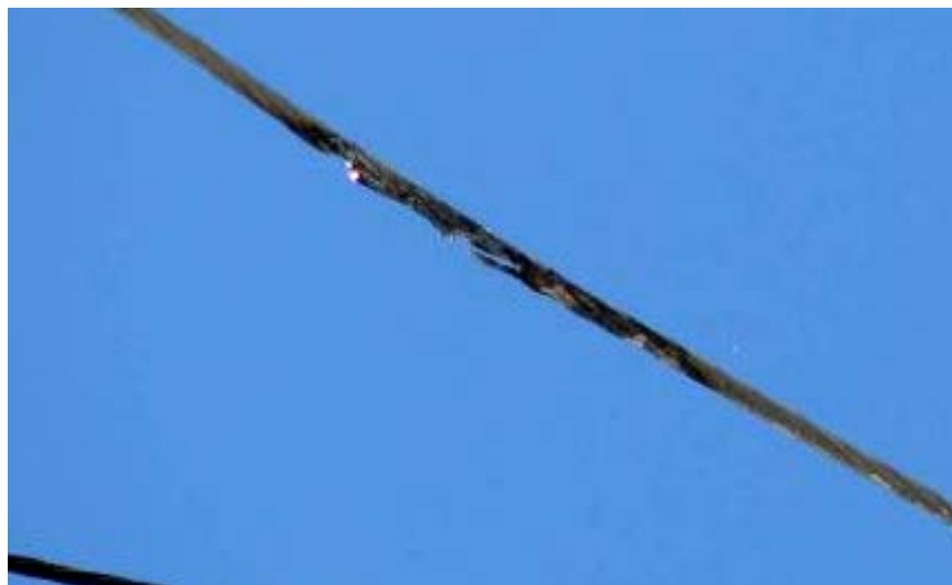
Figure 3-22 Photograph of Line Construction in Area of Wind-Induced Conductor Slap
