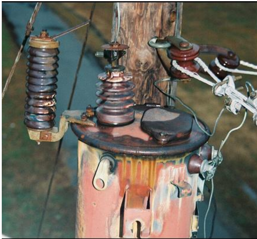
Figure 3-3 Transformer with Damaged External Bushing That Caused Intermittent Faults
