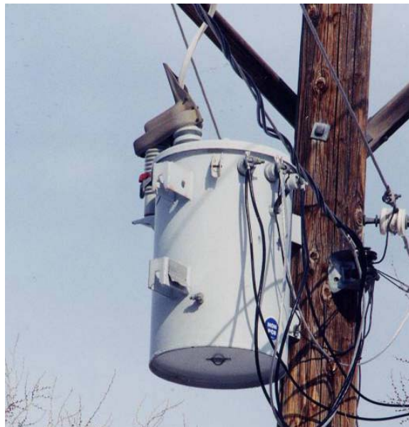
Figure 3-7 Combination Bushing and Arrester Cap
