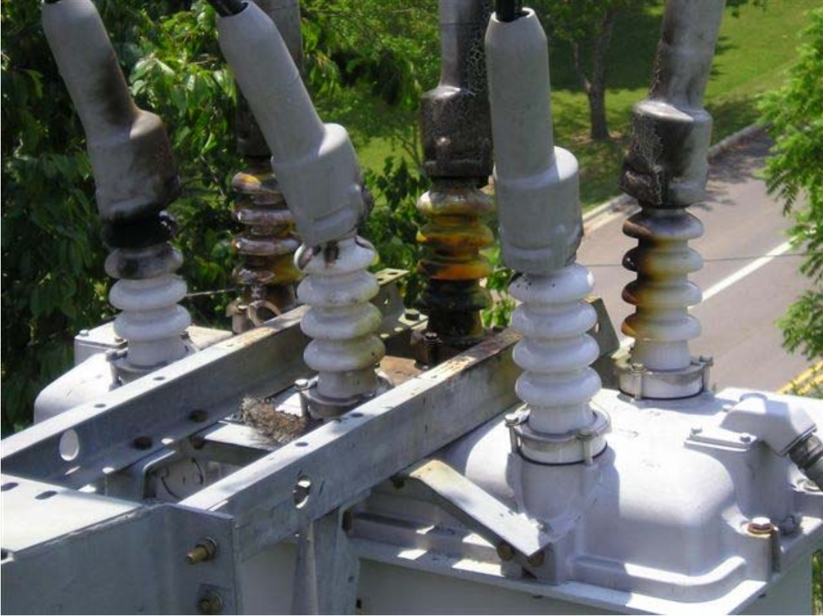
Figure 3-1 Poorly Fitting Wildlife Guards Do Not Mitigate Wildlife Interactions
