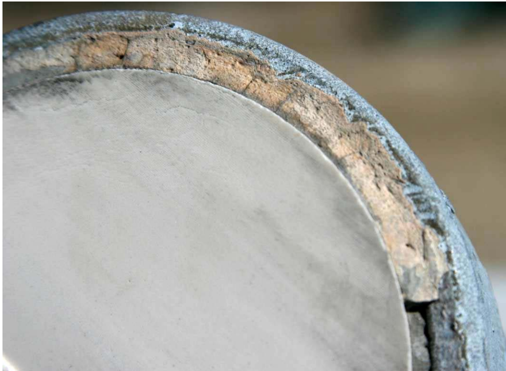
Figure 2-7 Cut Surface of Sample #2 Showing Cracks Near the Circumference of the Insulator
