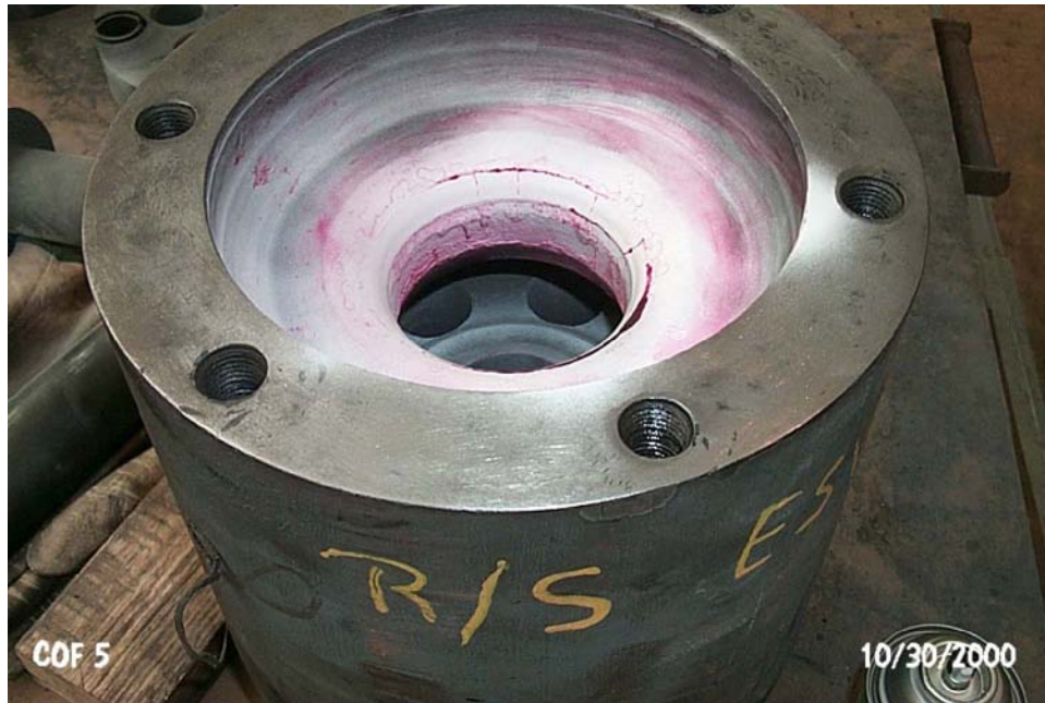
Figure 4-9 Stellite weld metal cracks in the bypass valve seat of an emergency stop valve
