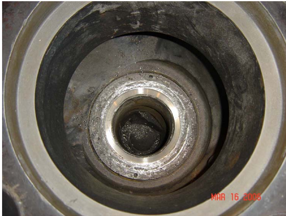
Figure 4-10 Machined weld prep for the control valve seat repair
