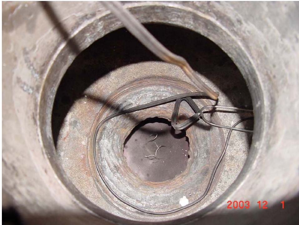
Figure 4-12 Weld-repaired seat for a Westinghouse governor valve
