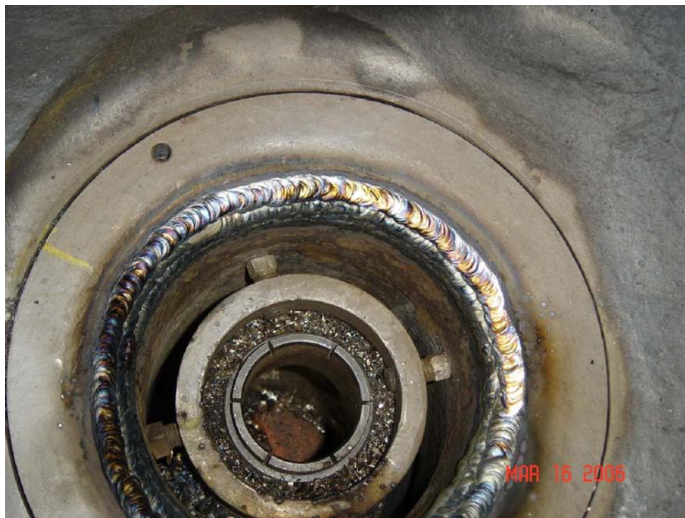
Figure 4-11 Weld repair beads on the control valve seat
