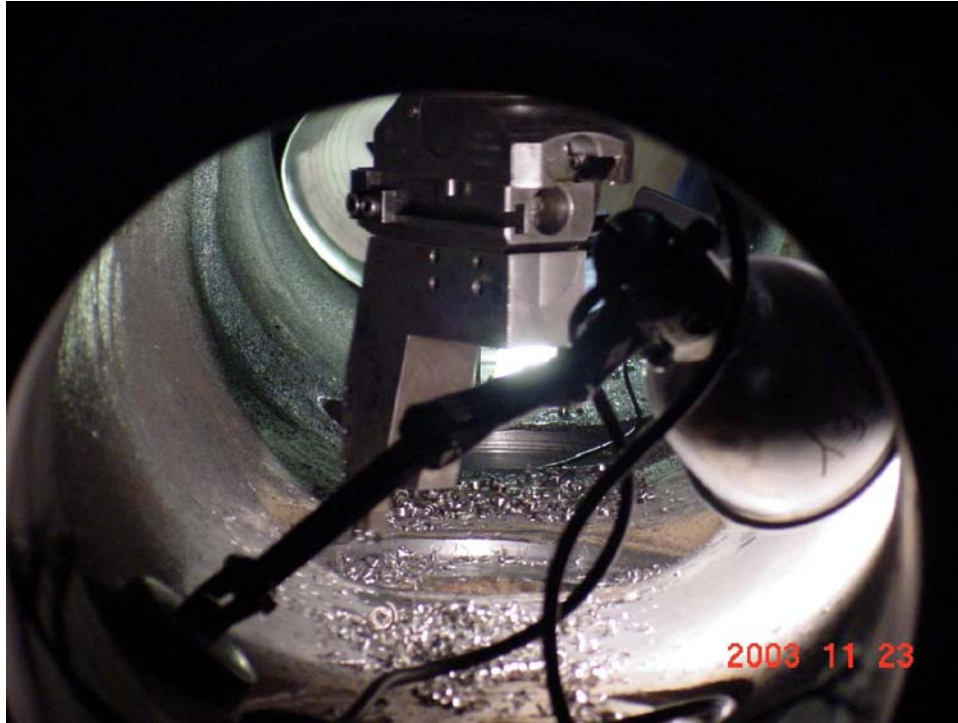
Figure 4-13 Machining of a governor valve seat
