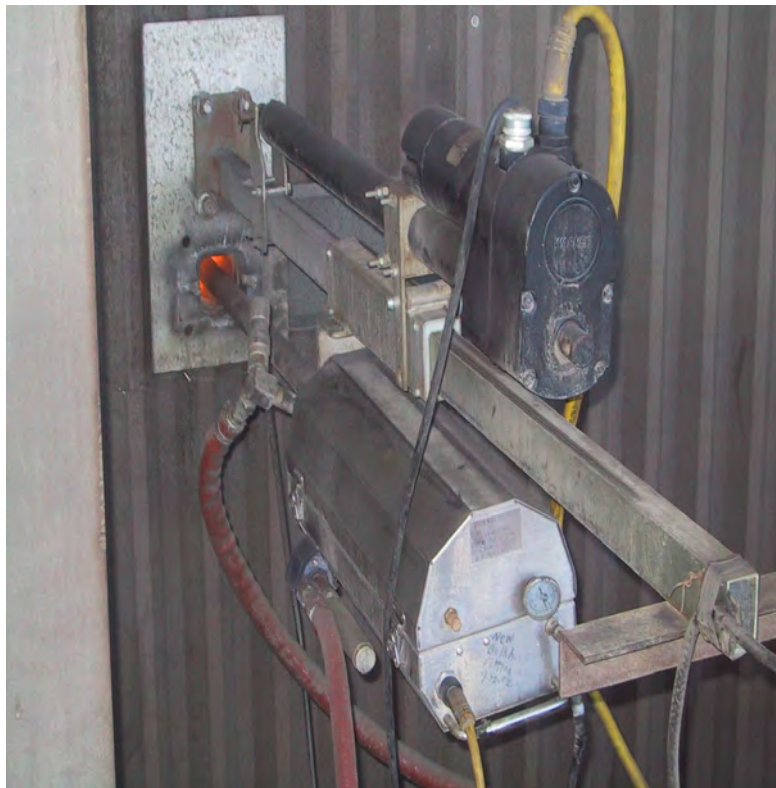
Figure 6-1 Diamond Power Flue Gas Temperature Camera
