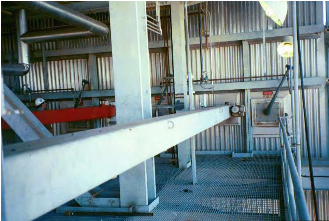
Figure 3-9 Three of Twelve Sonic Horns Installed in an Economizer through Existing Access Ports
