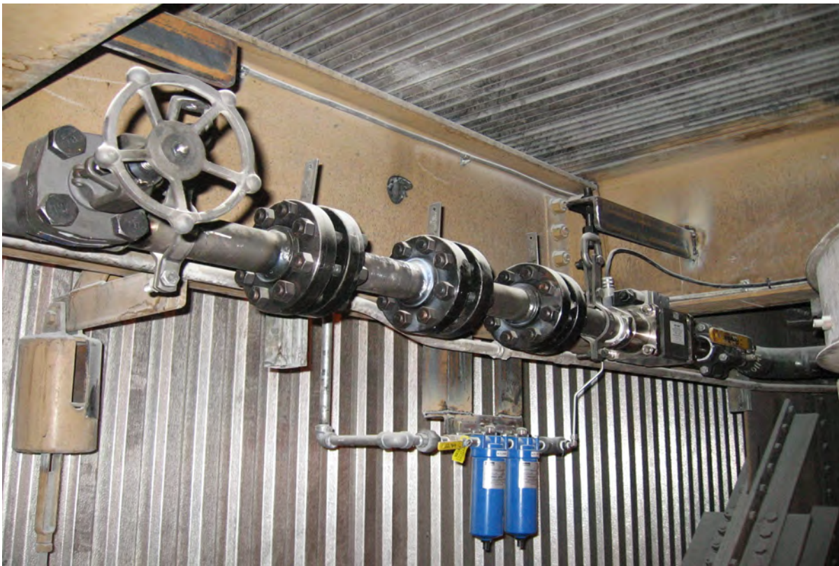
Figure B-1 Ring Header Recirculation Package for Water Hammer Control
