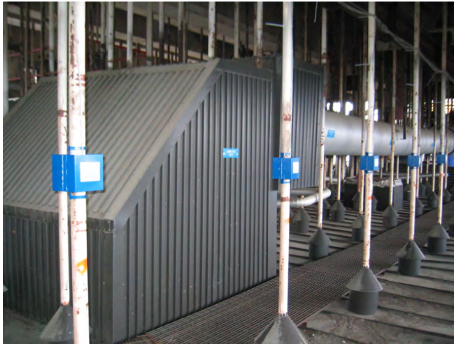
Figure 6-4 Strain gages on the Superheat Support Rods (20)
