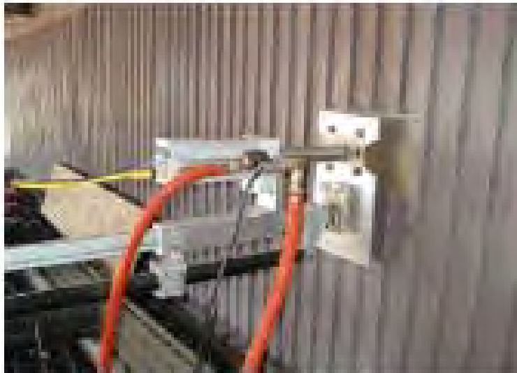
Figure 6-2 Diamond Power Gas Temp FEGT at TVA's Cumberland Plant
