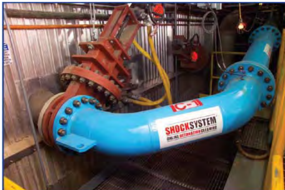
Figure 3-6 Photo of a Bent Tube SHOCKSystem Installed at AEP's Rockport Plant (6)
