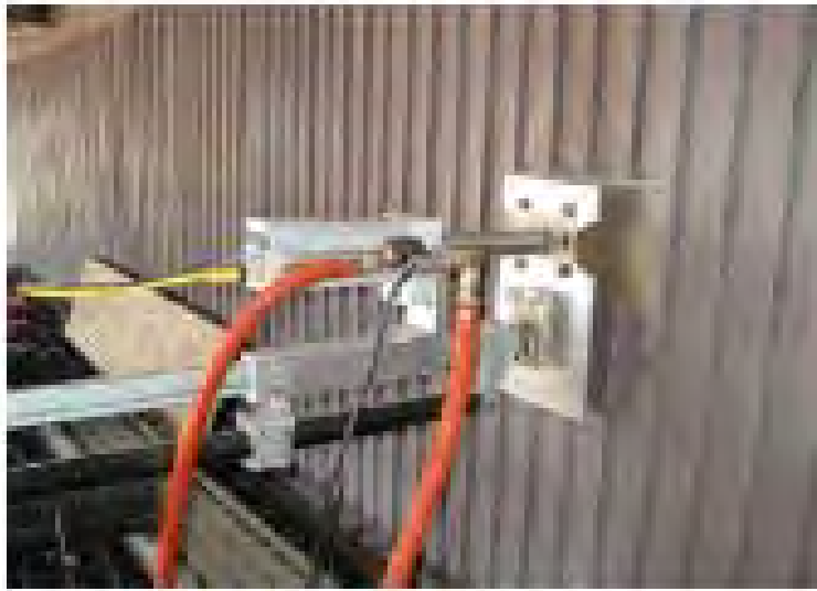
Figure 6-2 Diamond Power Gas Temp FEGT at TVA's Cumberland Plant
