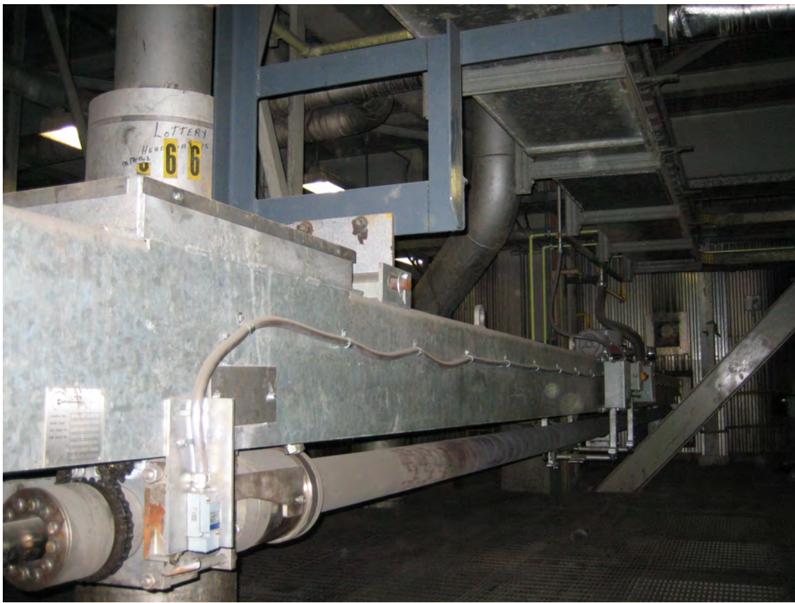
Figure 3-4 Photo of an Installed Multimedia Sootblower (Courtesy of Clyde Bergemann)
