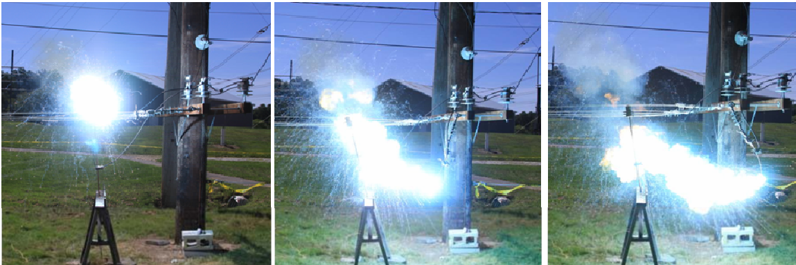
Figure 4-18 When the Conductor Breaks, the Energized End Swings Down, Pulling the Arc Out
