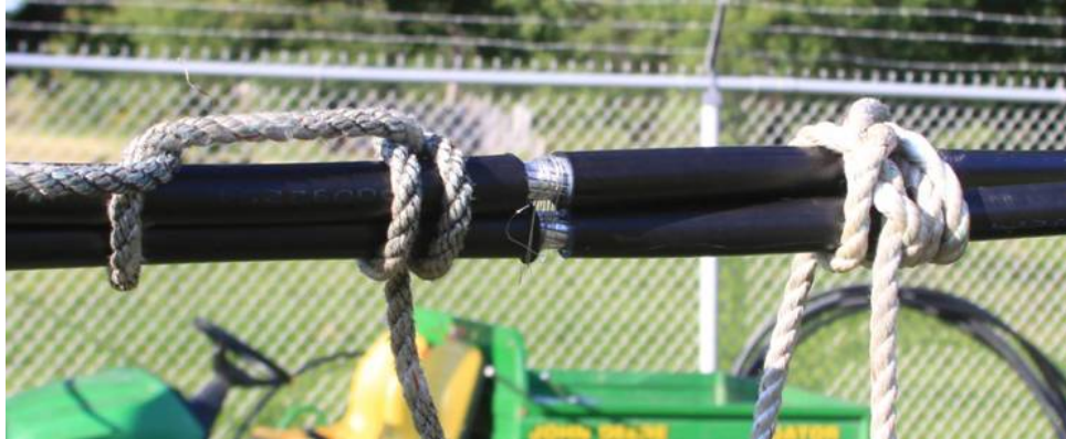
Figure 3-4 Test Configuration for Covered Conductors Tested at 8,700 Amps
