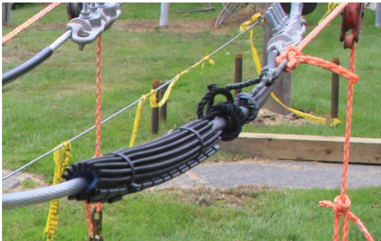
Figure 4-35 Gel Wrap Installed on a 336.4-kcmil (170.5-mm 2 ) Aluminum Conductor Prior to a Burndown Test
