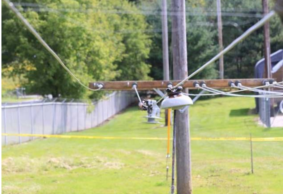
Figure 4-20 An Example of the Test Configuration Used for Arc Attachment Tests
